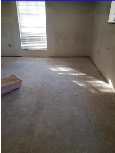
F. Item 1(Picture) Master bathroom
