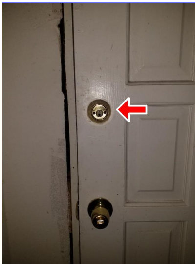
G. Item 3(Picture) Front door
