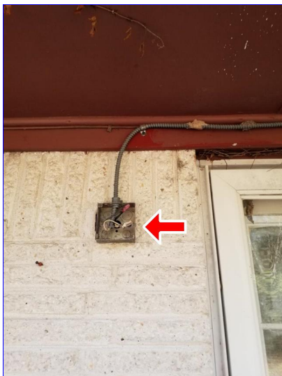
B. Item 1(Picture) Rear of home
