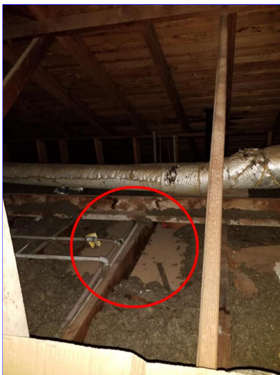
D. Item 3(Picture) Attic, front of home
