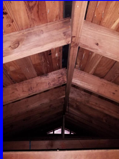
Roof structure stick built with wood slats
