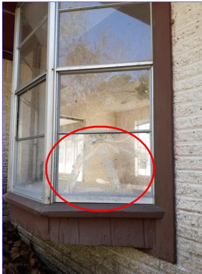
H. Item 9(Picture) Rear of home
