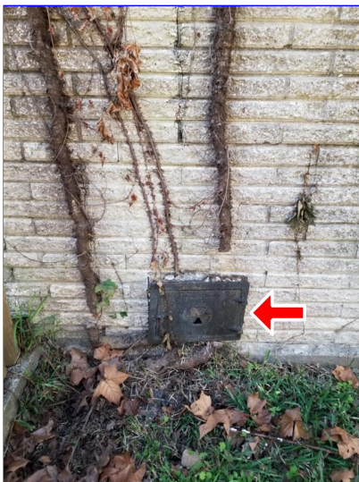
J. Item 1(Picture) Rear of home
