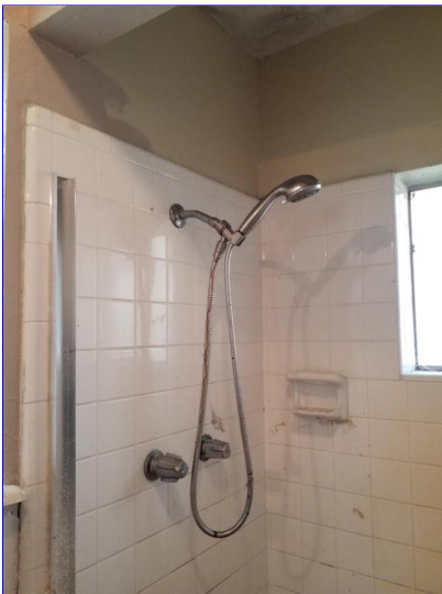
A. Item 3(Picture) Master bathroom
