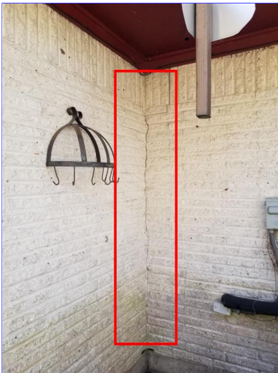
E. Item 23(Picture) Rear of home
