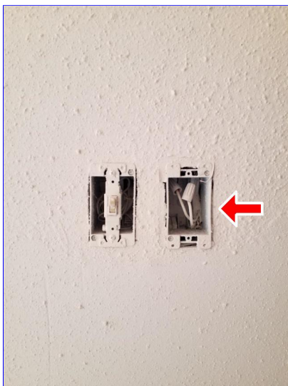
B. Item 3(Picture) Hallway in-between guest bedrooms
