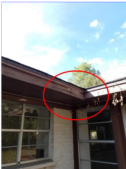
E. Item 14(Picture) Rear of home
