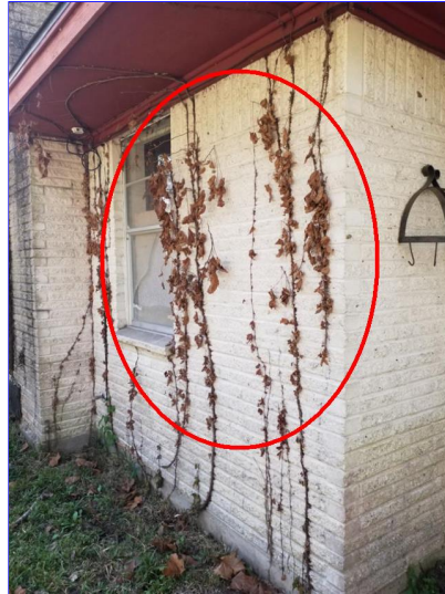
E. Item 5(Picture) Rear of home
