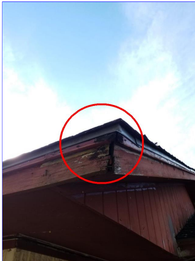
E. Item 16(Picture) Rear of home
