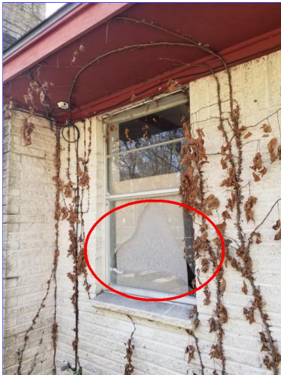
H. Item 8(Picture) Rear of home
