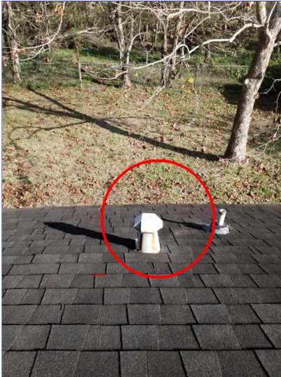
C. Item 5(Picture) Rear of home
