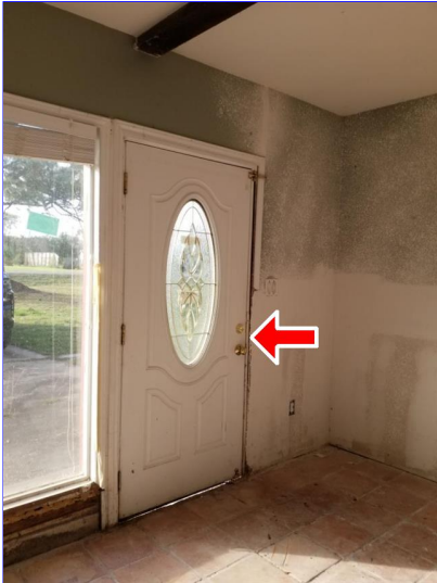
G. Item 1(Picture) Media room
