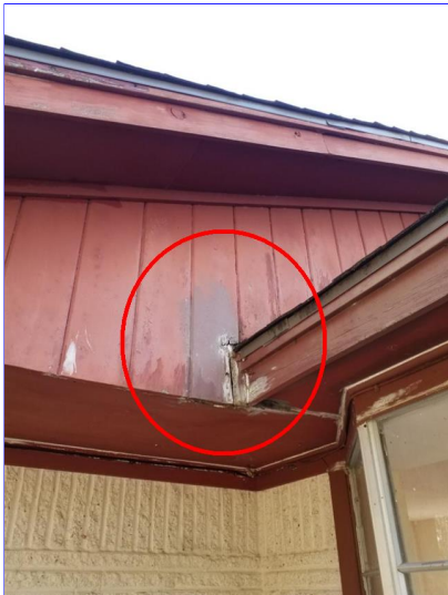
E. Item 15(Picture) Rear of home
