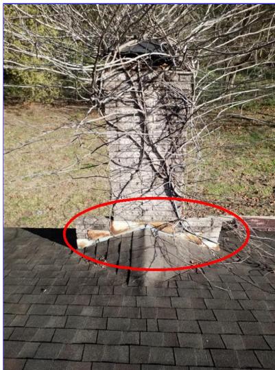
C. Item 2(Picture) Rear of home
