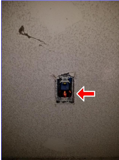
B. Item 10(Picture) Front entry, behind the front door
