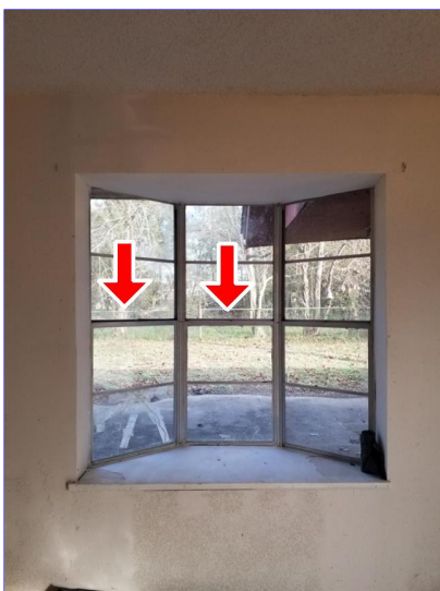
H. Item 11(Picture) Dining room, left and middle window
