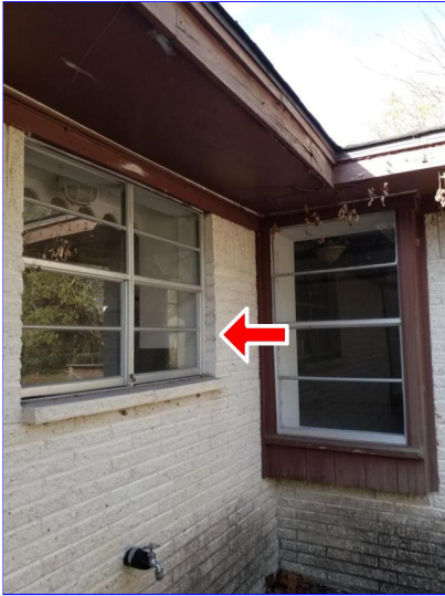
H. Item 5(Picture) Rear of home
