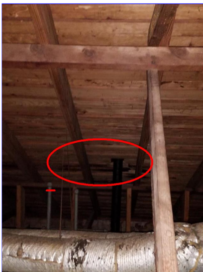
D. Item 4(Picture) Attic, front of home
