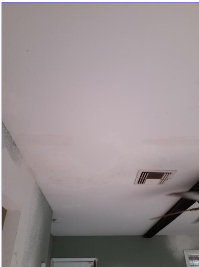
F. Item 2(Picture) Media room
