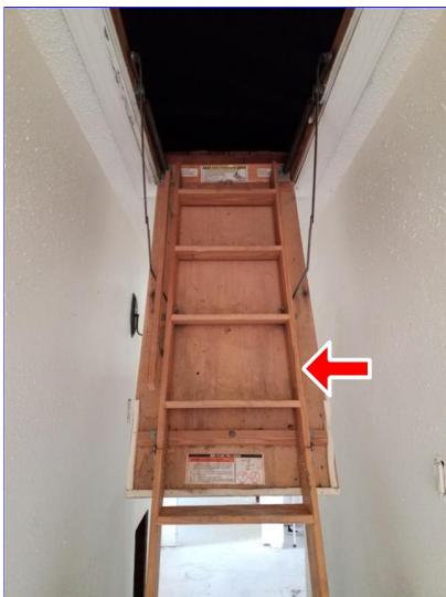
D. Item 1(Picture) Attic stairs
