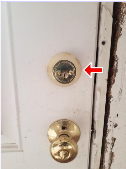
G. Item 2(Picture) Media room
