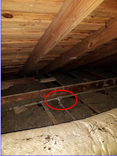
A. Item 4(Picture) Attic, rear of home
