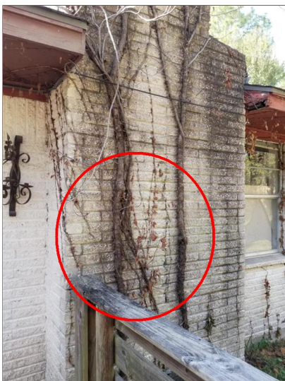
J. Item 2(Picture) Rear of home
