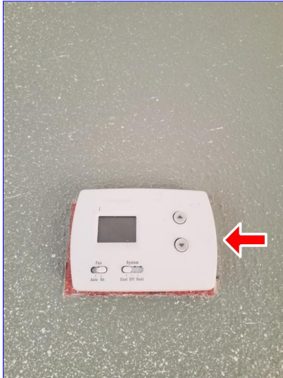
B. Item 1(Picture) Unit #2 (right side of home)
