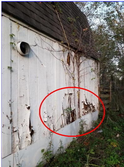
C. Item 4(Picture) Right side
