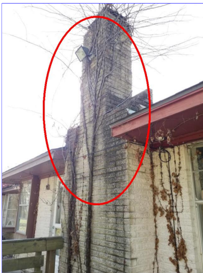
E. Item 6(Picture) Chimney
