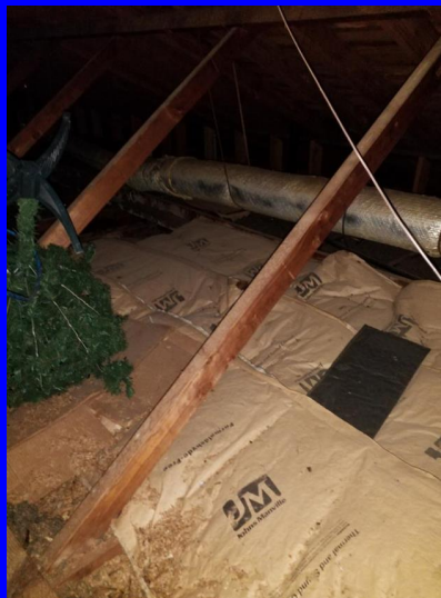
Less than six inches of batt fiberglass and rock wool insulation
