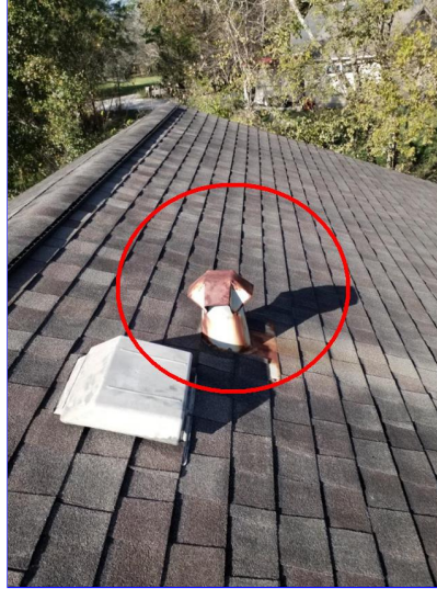
C. Item 4(Picture) Rear of home
