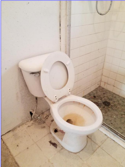
A. Item 1(Picture) Master bathroom
