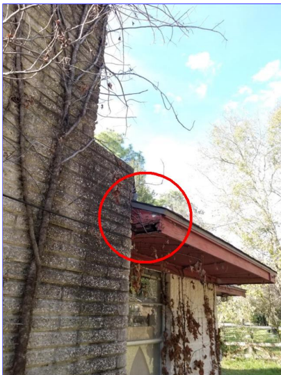
E. Item 17(Picture) Rear of home
