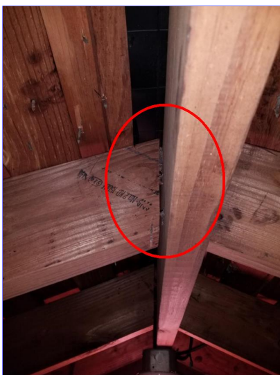
D. Item 2(Picture) Attic
