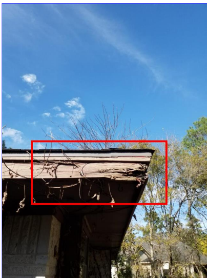
E. Item 13(Picture) Rear of home
