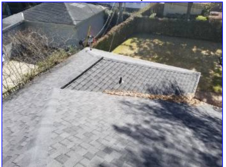
All visible roofing materials appeared to be properly installed at time of inspection.
