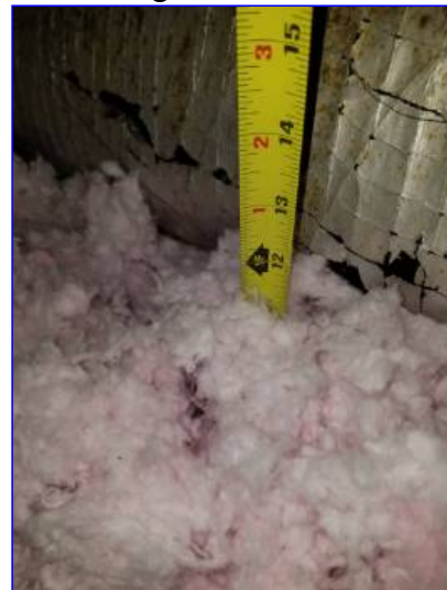
Insulation in the attic was measured at 10-12 inches.
