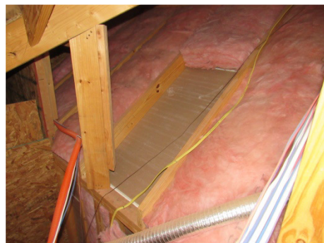
Missing insulation
