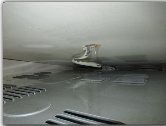
The 220 outlet box for the range was not secured to the wall.
