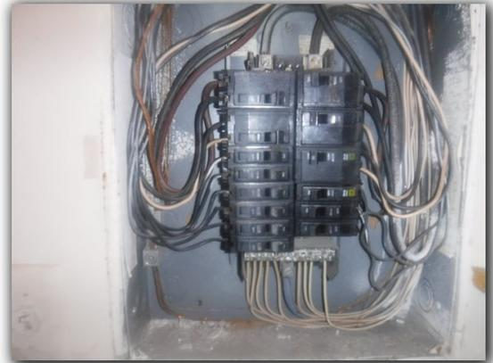
All panels are located in the closet across from the main entries of all units. Electrical panels are code required to not be behind any door that can lock and should be accessible to all occupants.
