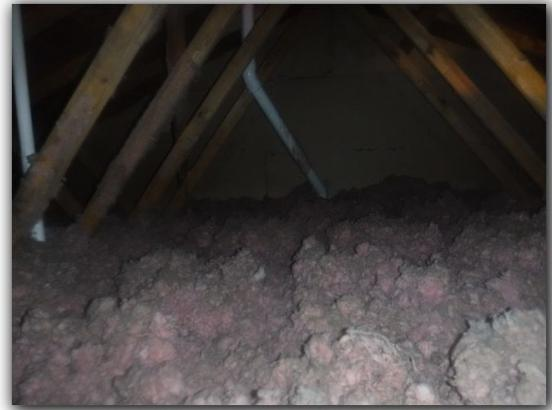
Insufficient attic insulation. Current code requires 13 inches of insulation for an R factor of 38.
