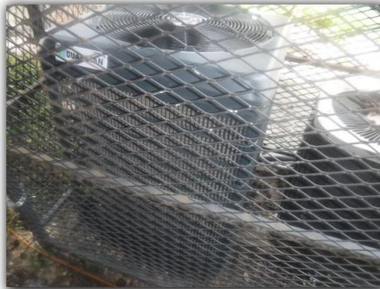
Supply air Temp 50 F    Return air Temp 73 F    Temp. Differential 23
