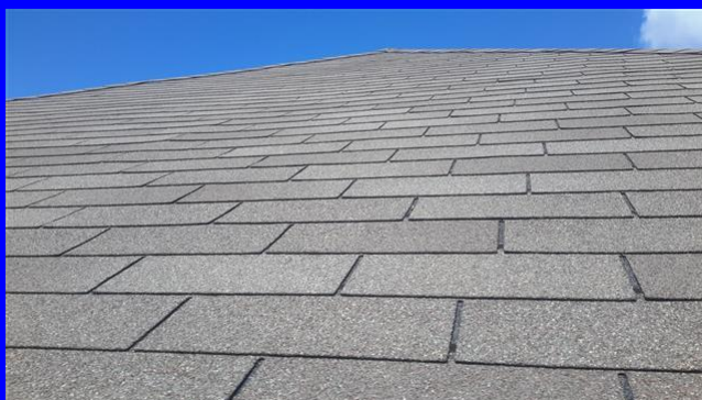
Roof overview, back
