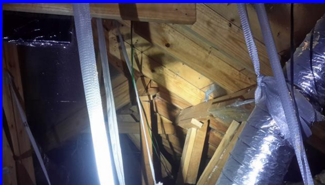
Stick built 2x6 rafters with TechShield
