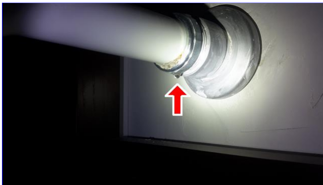
B. Item 2(Picture) 1st floor powder room
