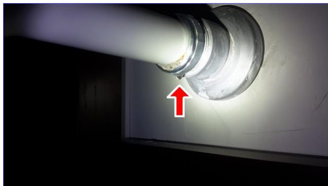
B. Item 2(Picture) 1st floor powder room
