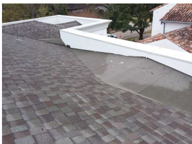
Viewed From: Walked Accessible Areas
