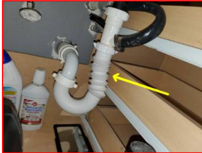
Flex drain pipes are not recommended because they can enhance clogs.
