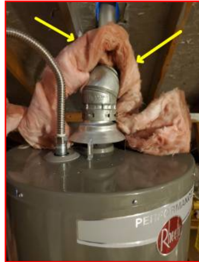
Insulation should not be touching exhaust pipe.
