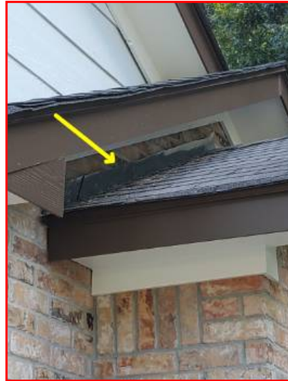
Flashing not installed correctly.
