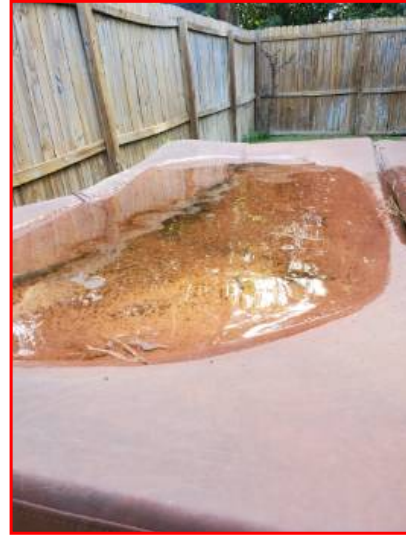
Top was damaged and holding water.
