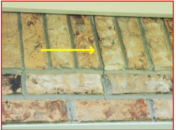
Cracks were noted.
