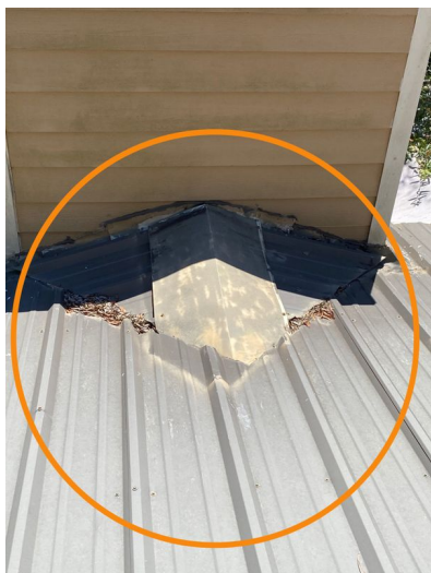
Front Exterior Wall
