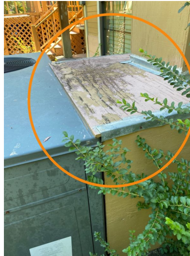
Right Exterior Wall
