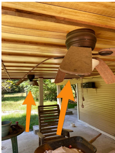
Example Left Exterior Wall
