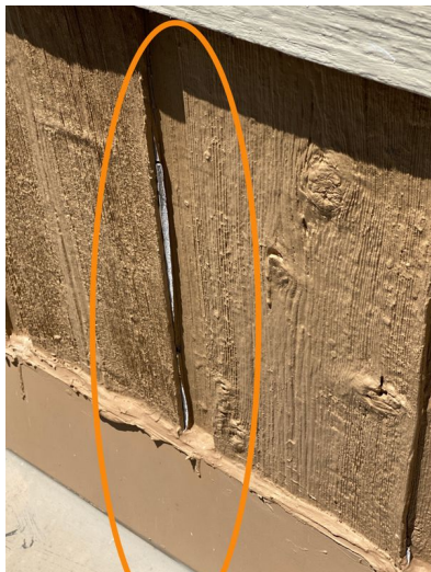
Front Exterior Wall
