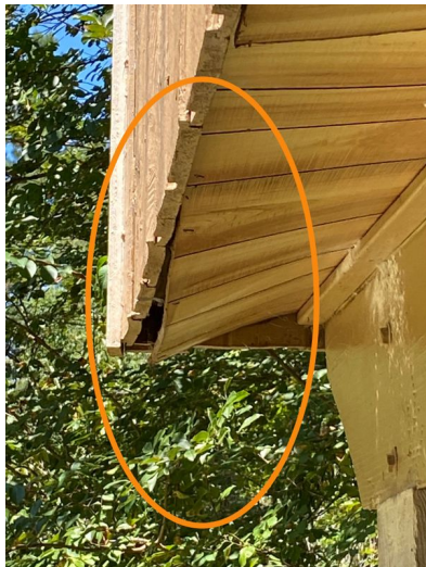
Example Left Exterior Wall
