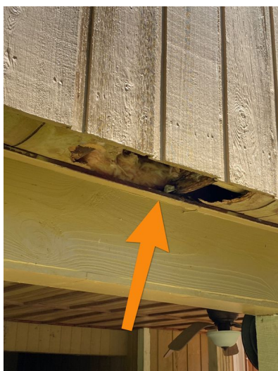
Example Left Exterior Wall
