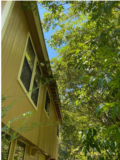
Example Rear Exterior Wall
