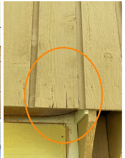
Example Rear Exterior Wall
