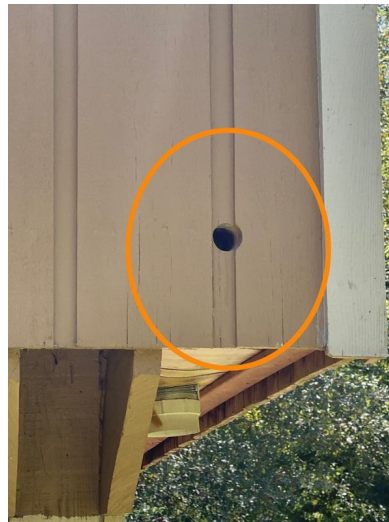
Example Rear Exterior Wall
