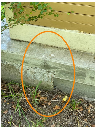
Example Rear Exterior Wall
