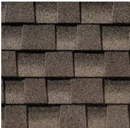
Roof. Weathered Wood Per Community Guidelines
