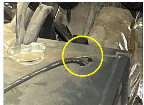
Electrical wiring not secured, the unit in attic.
