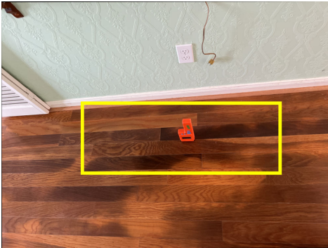
Water damaged wood flooring observed in the foyer. Moisture meters registered a 20.3 showing the area was active (wet).
