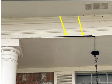
Observe large gap in the ceiling above the front door recommend repair to prevent rodent entry.
