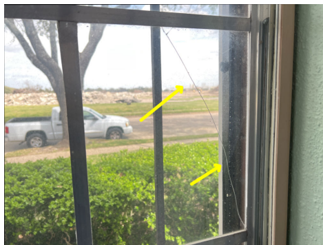
Crack window observed in the study.
