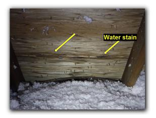
Observed older style roof framing in the attic. This type of framing was common practice at the time of construction, but would not be up to current standards.
