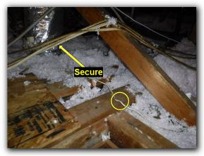
Observed one or more nails/screws missing from attic access ladder frame. Recommend installing a 16d nail or 1/4 inch diameter lag screw to properly secure stairway frame to ceiling.
