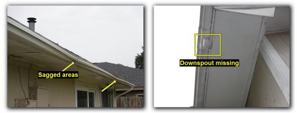
One or more splash blocks missing. Recommend adding splash blocks to divert water away from the foundation.
