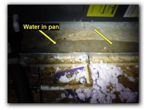
The primary drain line does not appear to be trapped. Current standards call for the primary drain line to be trapped (it is possible the trap is buried in insulation).
