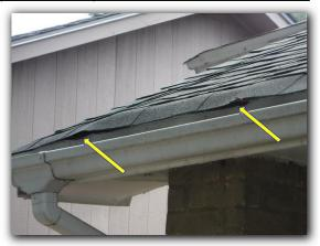
Observed siding touching shingles in one or more areas of roof. Common industry practice calls for at least a two inch separation from bottom edge of siding and roof surface. The two inch separation helps prevent moisture from being trapped which can cause deterioration.
