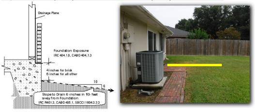
Observed soil levels too high around the foundation in one or more areas. High soil levels are considered a conducive condition to termite activity and water penetration.
