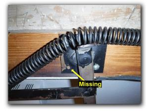
Observed loose hardware on the attic access ladder. Recommend tightening as needed.
