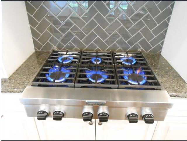
D. Item 4(Picture) View of the cooktop functioning.
