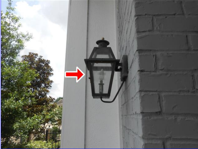
B. Item 2(Picture) This light failed to light with activation of the light switch.
