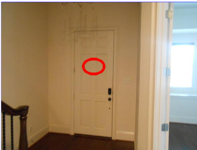
G. Item 2(Picture) Install peep hole
