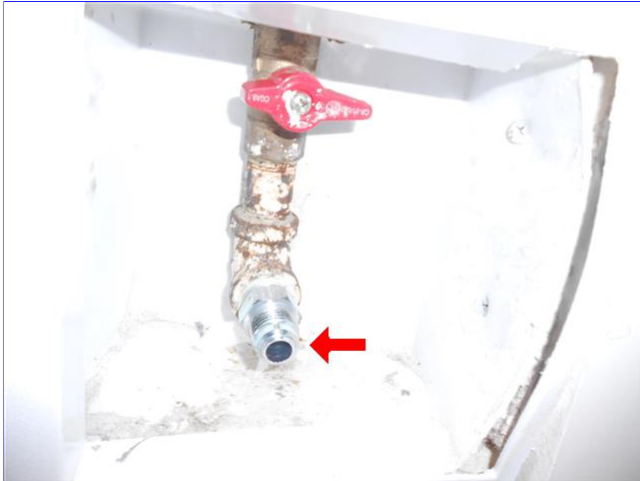
L. Item 1(Picture) Unused gas valves need to be capped
