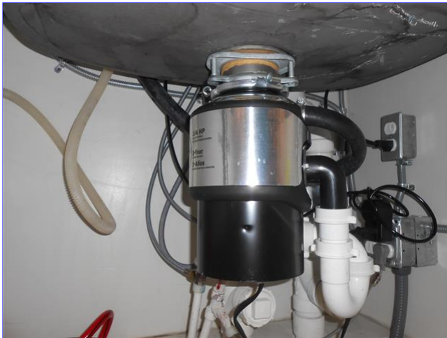
B. Item 1(Picture) View of the Food Waste Disposer
