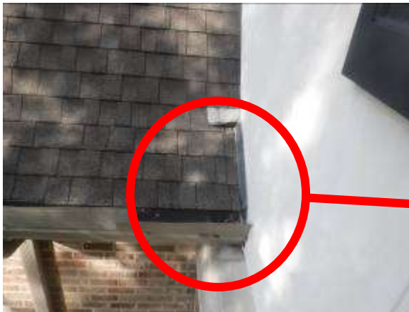
Missing kickout flashing
