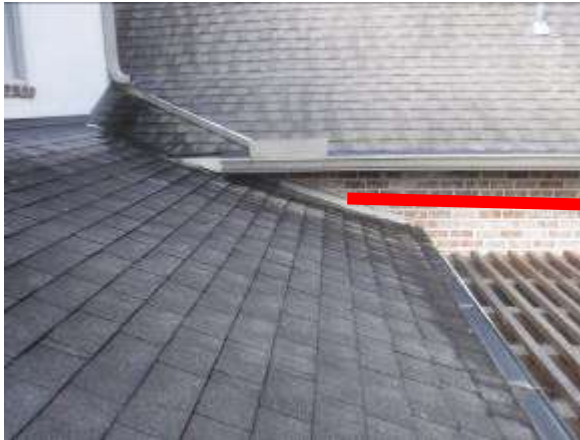
Rear of the house
