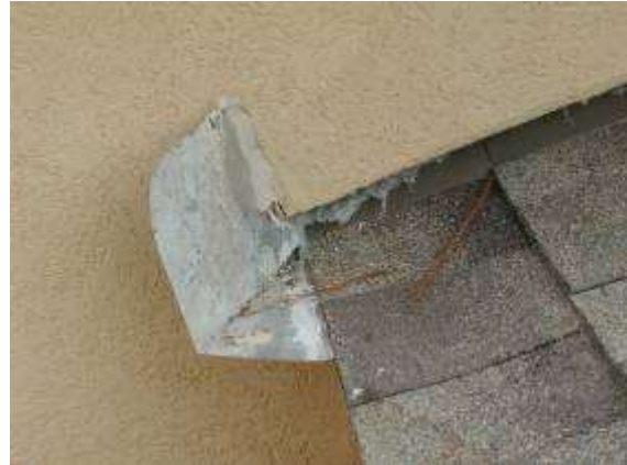
HEI file photo illustrating kickout flashing
