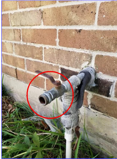
A. Item 2(Picture) Front left side of home
