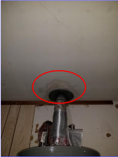
F. Item 1(Picture) Garage
