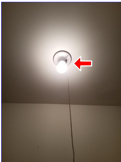
B. Item 9(Picture) Guest bedroom closet, on the left
