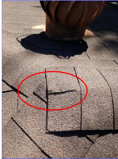
C. Item 7(Picture) Front of home
