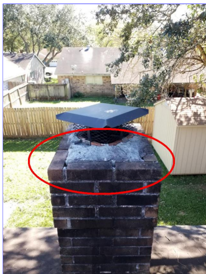
J. Item 3(Picture) Chimney
