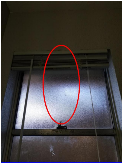
H. Item 12(Picture) Master bathroom
