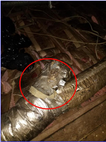
C. Item 2(Picture) Attic
