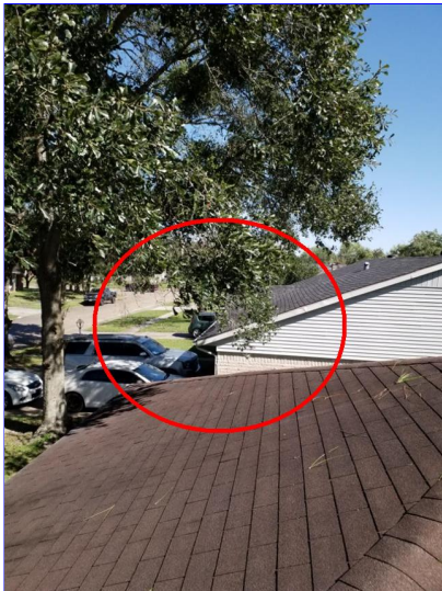
C. Item 5(Picture) Front of home
