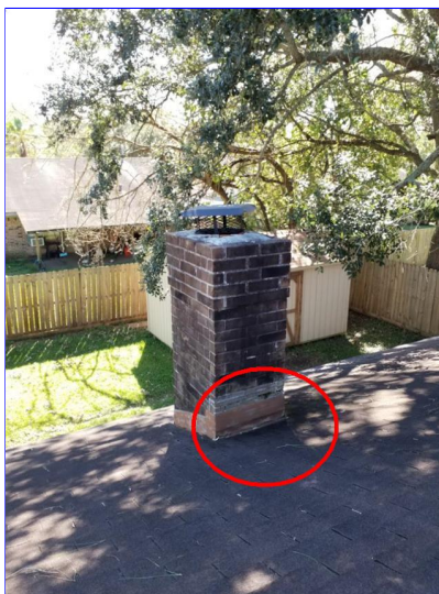
J. Item 2(Picture) Chimney
