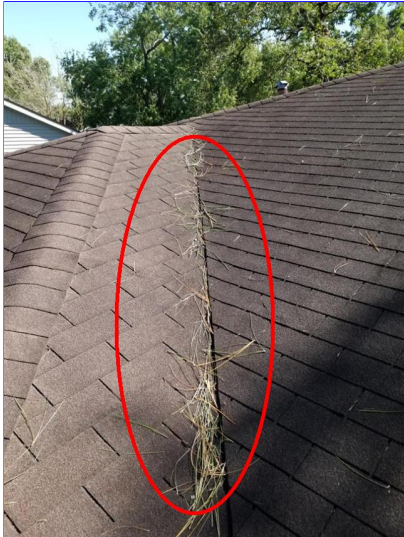
C. Item 4(Picture) Front of home
