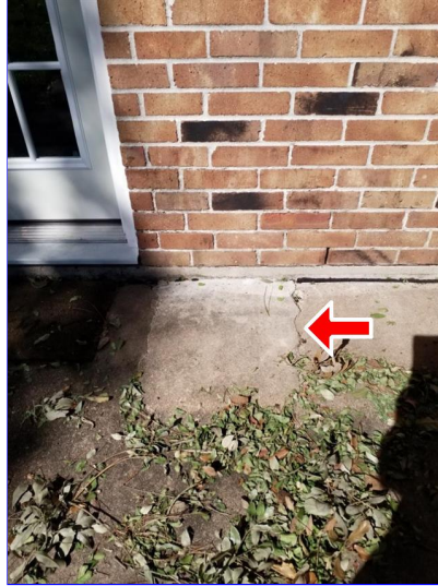
A. Item 6(Picture) Rear of home
