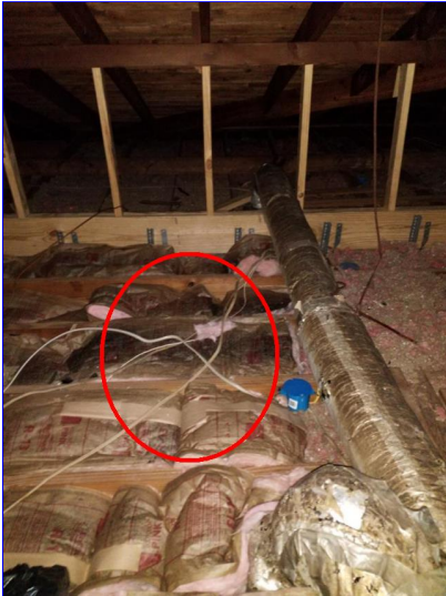
B. Item 13(Picture) Attic
