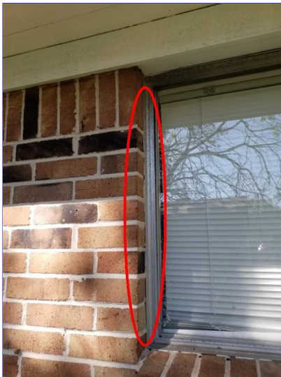
H. Item 9(Picture) Rear of home
