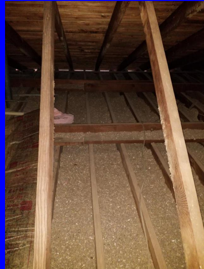
Less than six inches of cellulose insulation
