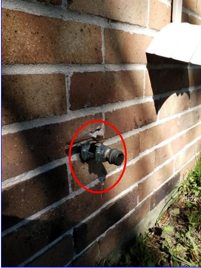
A. Item 4(Picture) Rear of home
