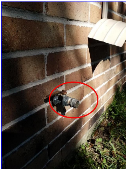
A. Item 3(Picture) Rear of home
