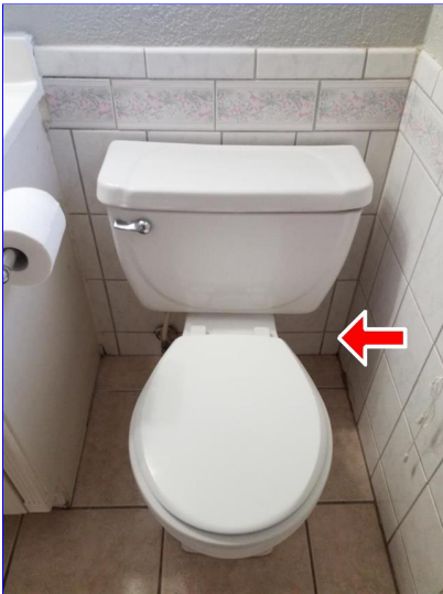
A. Item 5(Picture) Master bathroom, runs continuously
