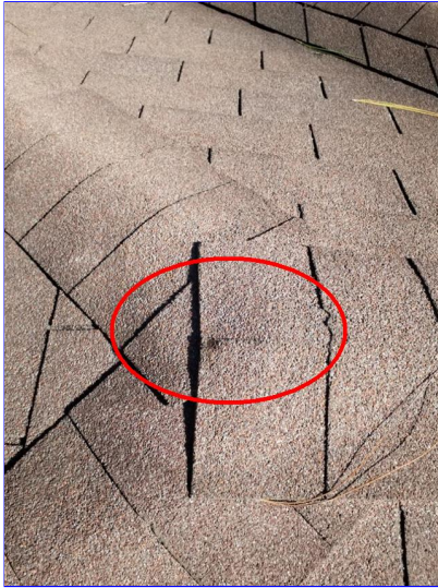
C. Item 6(Picture) Front of home
