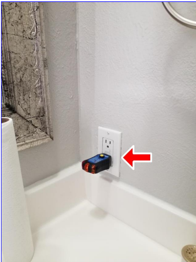
B. Item 7(Picture) Guest bathroom
