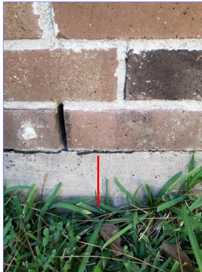
A. Item 8(Picture) Left side of home
