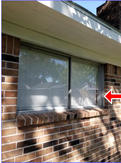
H. Item 6(Picture) Rear of home
