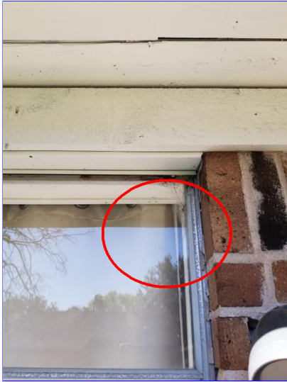
H. Item 10(Picture) Rear of home
