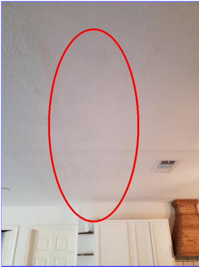
F. Item 3(Picture) Kitchen
