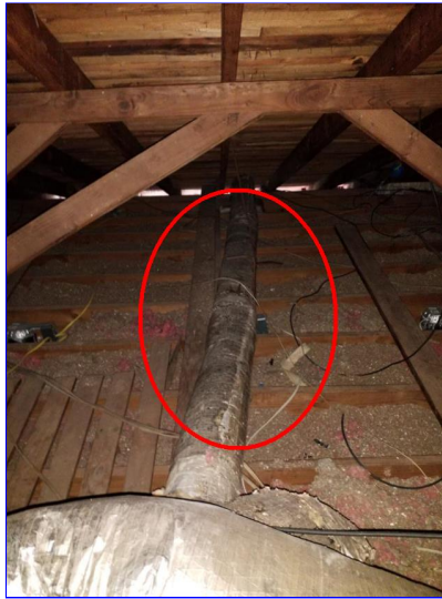
C. Item 3(Picture) Attic
