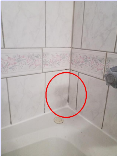
E. Item 12(Picture) Master bathroom
