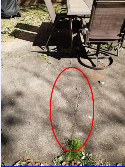
K. Item 1(Picture) Rear patio
