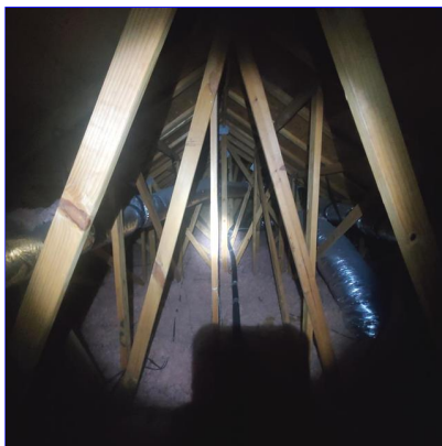
D. Item 2(Picture) General view of attic.
