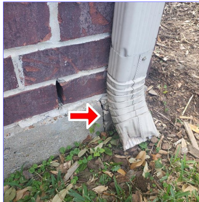
A. Item 4(Picture) Corner pop at the northwest corner of the home
