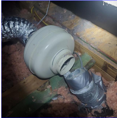
H. Item 2(Picture) Booster is fan loose in the attic and dryer is venting into the Attic
