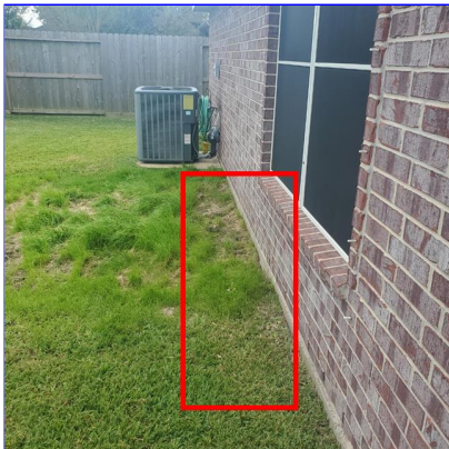
B. Item 3(Picture) Area for potential ponding water at the back of the home
