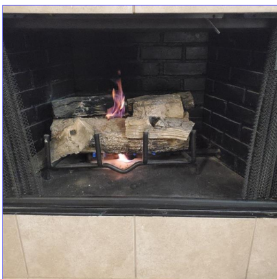
J. Item 3(Picture) General view of fireplace
