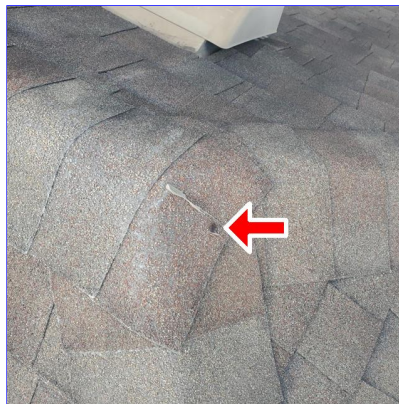
C. Item 4(Picture) Expose nails on ridge on the back facet of the home
