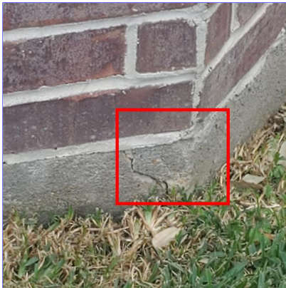
A. Item 3(Picture) Corner pop at the north side of the home
