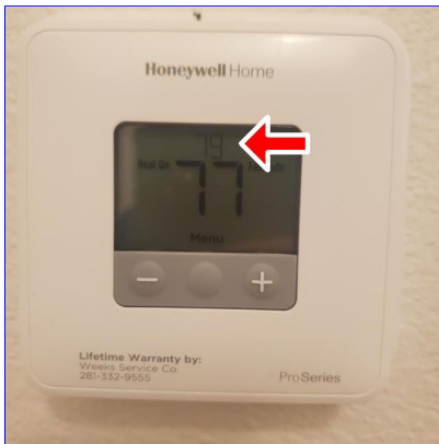
A. Item 1(Picture) The furnace was set to 79 degrees but would not come on and eat the home
