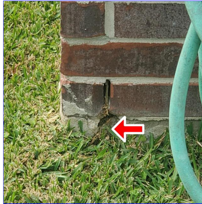
A. Item 2(Picture) Corner pop at the southeast corner of the home
