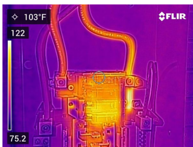
General Photos of Grounding System(s):
