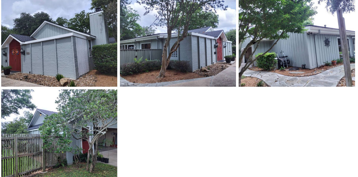
General Photos of Roof Covering:
