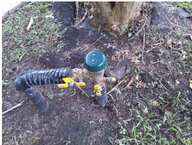
Vacuum Breaker/Backflow Preventer: Installed
