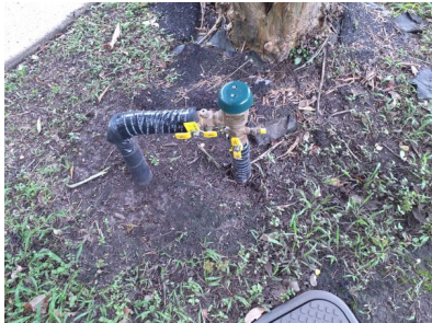
Vacuum Breaker/Backflow Preventer: Installed
