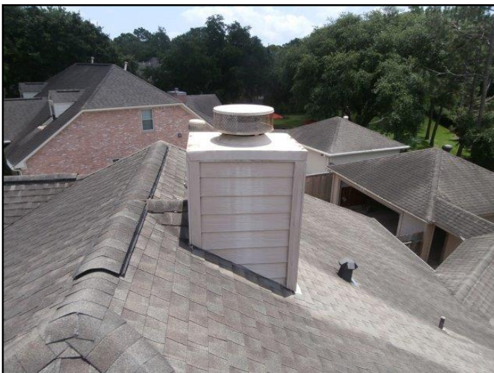
General view of roof covering.
