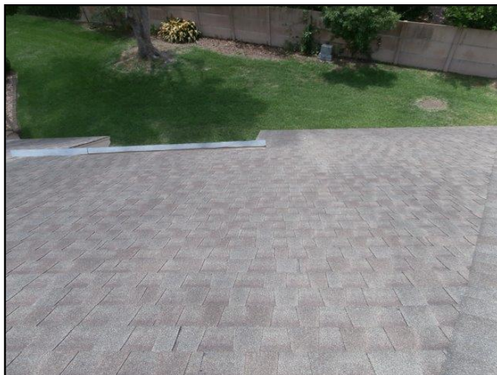
General view of roof covering.
