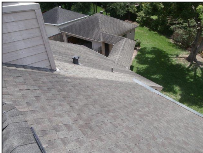
General view of roof covering.
