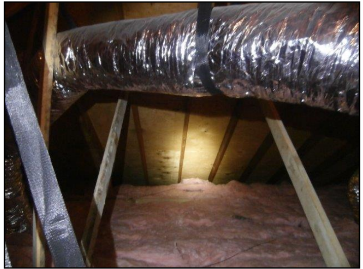
General view of attic structure.
