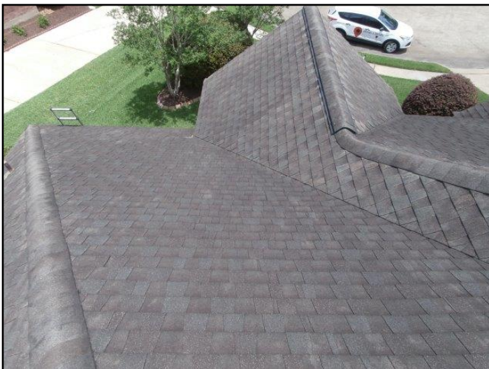
General view of roof covering.
