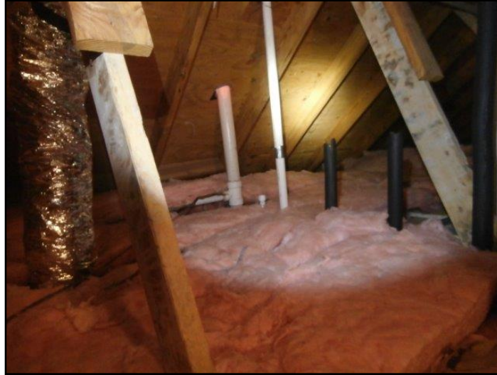
General view of attic insulation.
