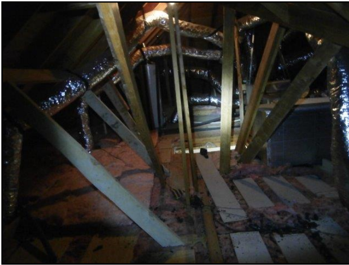
General view of attic structure.
