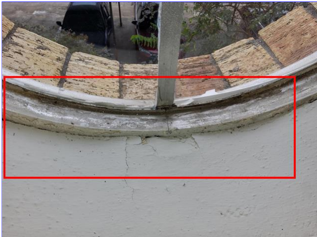
E. Item 6 (Picture) Main entry window
