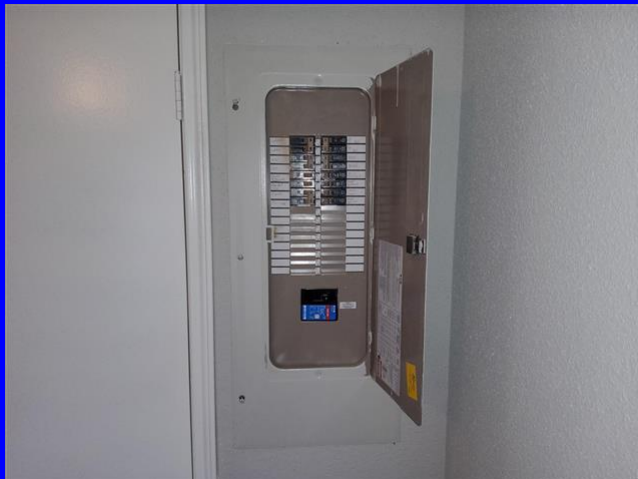
Eaton /Cutler Hammer service panel with 100 amp service
