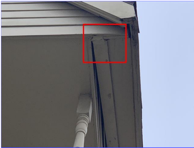
E. Item 13 (Picture) Balcony area
