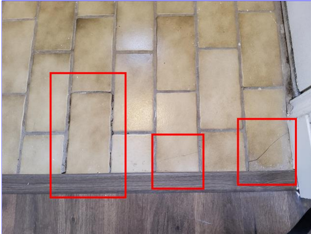
F. Item 1 (Picture) Main entry landing
