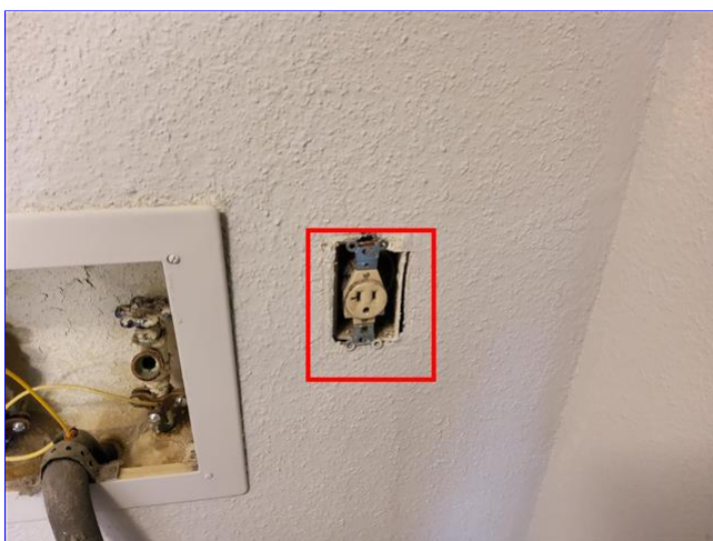
B. Item 4 (Picture) Laundry Room
