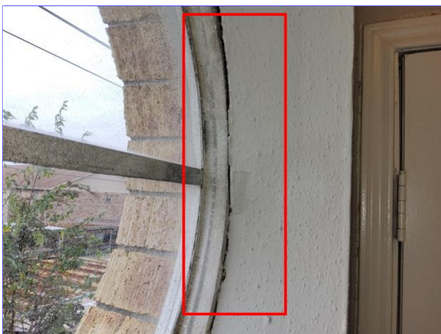
E. Item 7 (Picture) Main entry window
