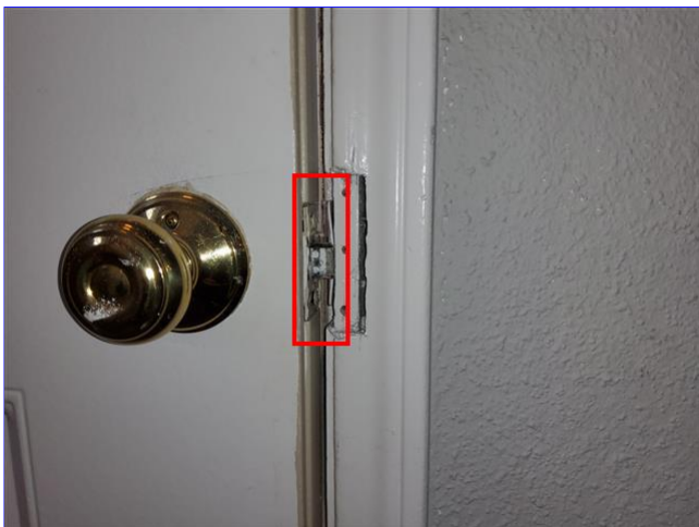
G. Item 1 (Picture) Main entry door.
