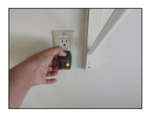
Outlet(s) found to be worn, does not hold the plug securely, recommend replacement, including but not limited to; in living room, some in master bedroom.
