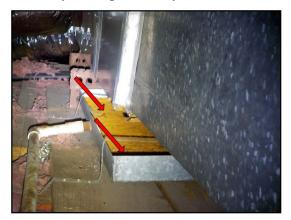
Emergency drain line/elbow observed to be broken over window.
