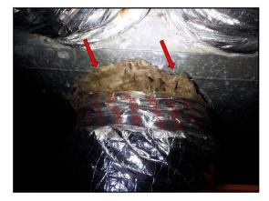
Some flex duct observed to be routed improperly, not to manufacturer's installation instructions. Recommend additional support and/or routing ducts to eliminate "snaking" drooping or crimping of flex duct more than 1" per foot which adds unnecessary additional resistance.
