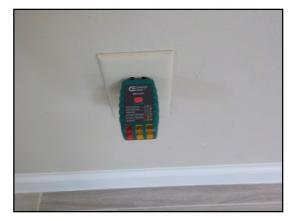
Improperly wired, 3 prong outlet not grounded or polarity reversed, including but not limited to; garage exterior,
