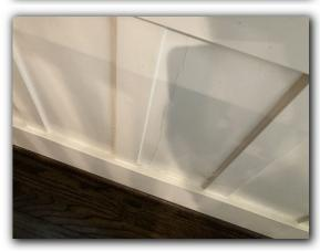
Separation was noted at sections of the interior trim and / or crown molding as evident of settlement of the structure.
