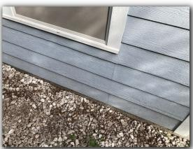
Waves / Waffling was noted at portions of the cement board siding.
