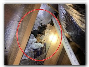
Voids were found at the water heater and / or furnace flue pipes as evident by daylight. Recommend repairs to prevent water penetrations.
