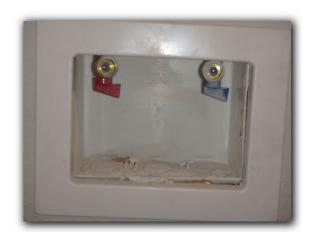
Hose Bibs: Anti siphon devices were installed. No deficiency was observed.
