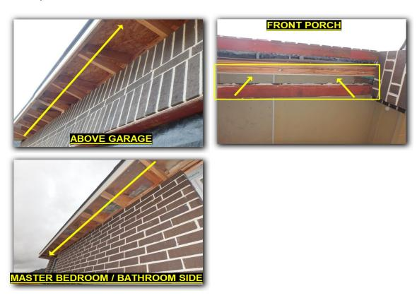
Flashing: All flashing to be painted, such as at window headers, and on roof coverings at drip edges, and at roof / wall joints.
