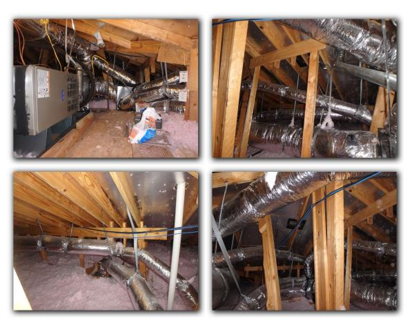
Attic was insulated with blowing fiber glass insulation which approximately measured 10+ inches that complies with the R30 insulation requirements.
