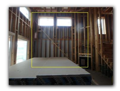
Wind storm brackets: The hurricane / wind storm brackets were not installed.
