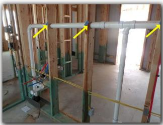
Nail plates: Gas pipes: Install nail plate in kitchen area.
