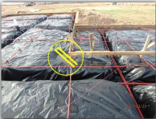
Standing water: Standing water was observed in most footings and also on slab areas, due to rain in early morning. Before foundation pour, the standing water should be allowed to be dried or should be pumped out.
