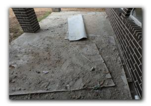
Drive Way: The drive way need to be cleaned. The concrete blocks could not be observed for cracks.
