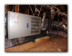
Number of Heating units: One, The unit was split in two zones, first floor zone and second floor zone.
