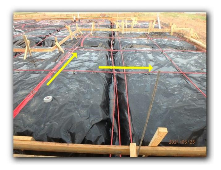
Plumbing drain pipes protection and chairs supports: Chair supports are required at all plumbing drain pipe locations. To be installed before the foundations pours.
