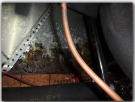
Secondary drain pan: The drain pan was significantly corroded. Also cool air was leaking from the front bottom edge near the primary drain pipe. To be further diagnosed and repaired by a licensed HVAC contractor.
