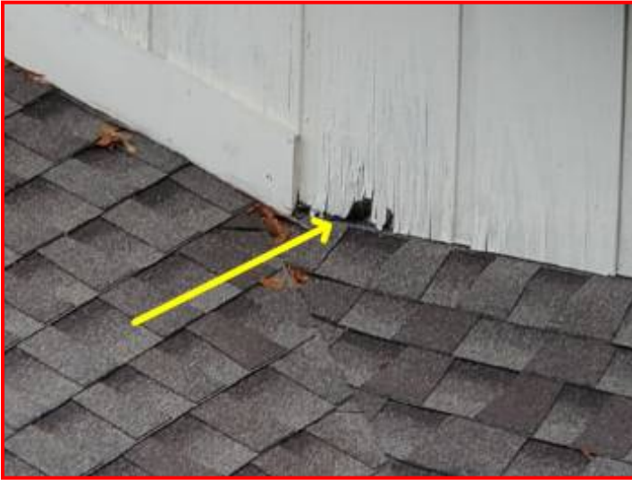
Damaged siding noticed in one or more areas.
