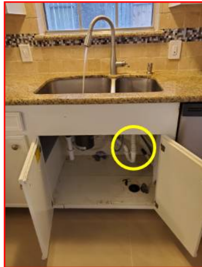
Flex drain pipes are not recommended because they can enhance clogs.
