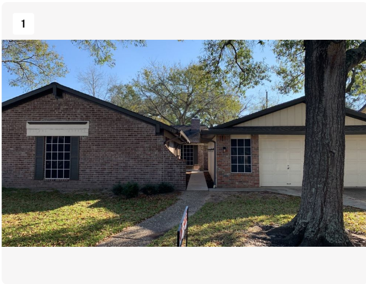
Overview -Front of Home
