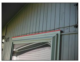
Head flashing missing over some windows / doors. Head flashing helps prevent water penetration. Without head flashing windows/ sealing must be maintained as the only defense against water penetration.
