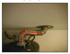
Not all double wall vent pipe connection(s) are properly secured together;
