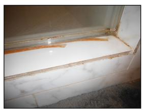
Grout / caulking needed at vertical tile corners, cracks in tile and/or mortar between tiles, to prevent water entry behind wall.
