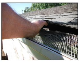
One or more areas of raised shingle tabs from fasteners not secured down properly or nail heads popping up through shingles.
