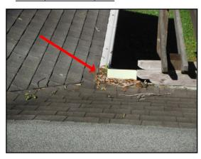
Downspouts need splash blocks at bottoms to prevent soil erosion.
