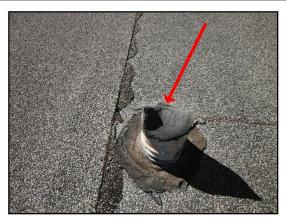
Painting of exterior plastic PVC vents above roof line required to prevent UV damage.
