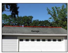
Exposed staples / nail heads / fasteners observed on roof are not properly sealed. Water entry possible.
