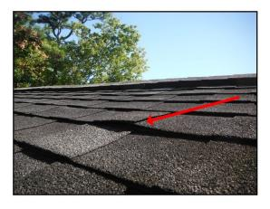
Roof tar repairs observed around roof penetration(s) and areas with missing flashing.
