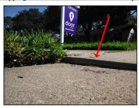
Rear patio has settled and has multiple cracks and uneven surface.
