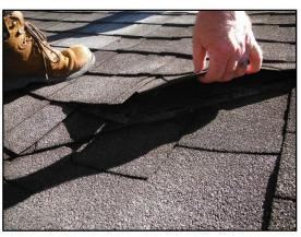
Improper installation of shingle starter course, not installed per manufacture's installation instructions on every bundle of shingle that instructs glue / sealing tabs to be located near lower edge of roofing. When starter course is not installed properly, high winds can peel roofing off. Reference: shingle bundle wrappers.
