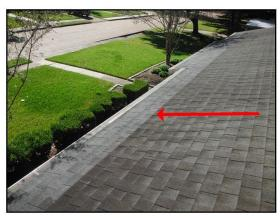
Valley shingles are installed improperly. Closed valley shingles are not embeded in roofing cement and/ or, the top corner is not clipped at a 45-degree angle. This prevents debris from getting caught in the shingles and accumulating in the valley, and also directs water toward the valley centerline.
