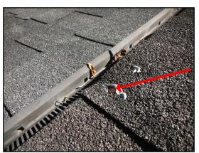
Older roof, nearing end of serviceable life. Observed Brittle, cracked, curled ends, and/or excessive granular loss of shingles.
