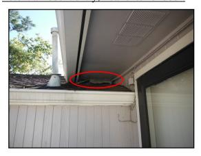
Need sealing / caulking around all holes and exterior siding penetrations on top and both sides, (*leave bottom open*) to prevent water entry. Including but not limited to dryer, bath and range top vents, light fixtures, etc.
