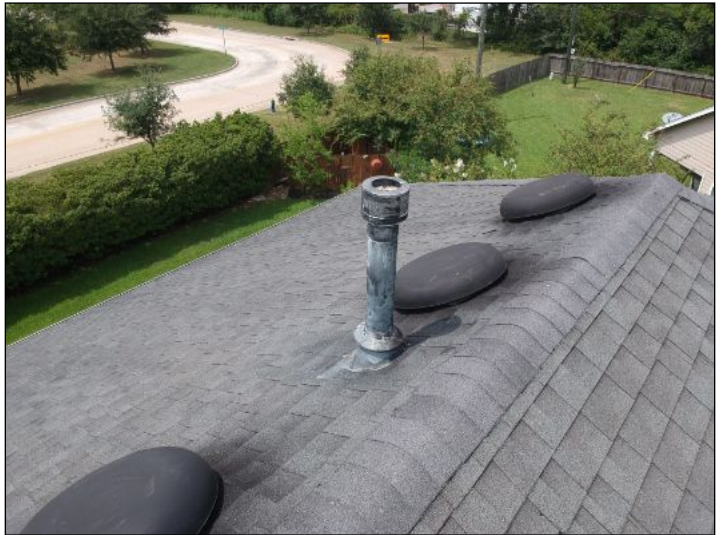
Overview of roof
