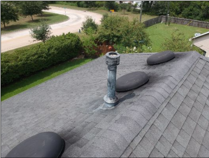
Overview of roof
