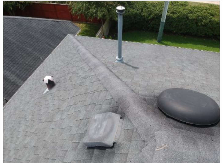
Overview of roof
