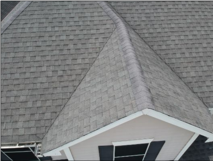
Overview of roof
