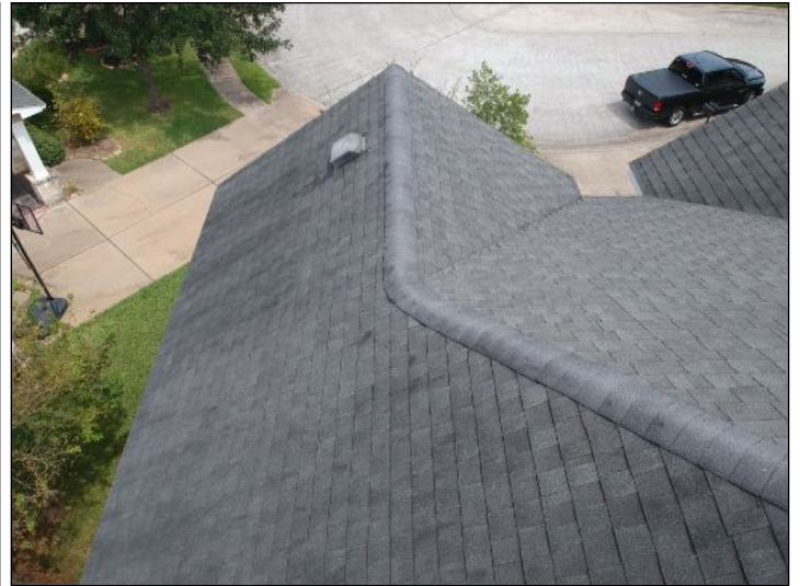
Overview of roof
