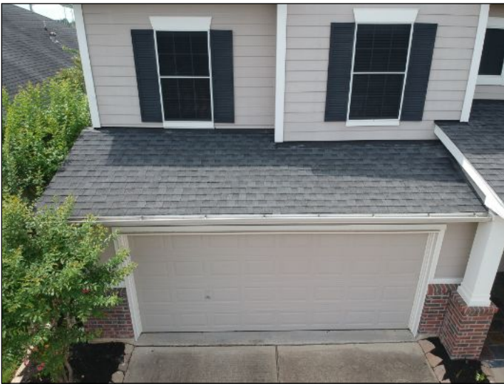
Overview of roof
