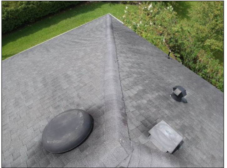
Overview of roof
