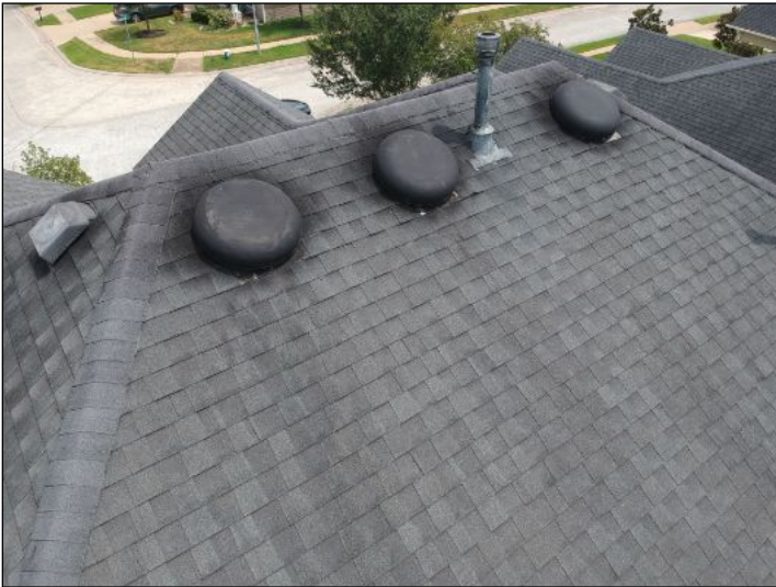
Overview of roof
