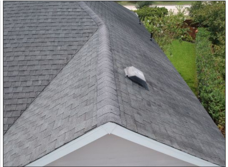
Overview of roof
