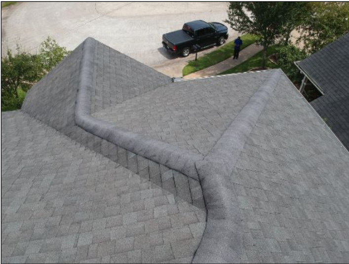
Overview of roof
