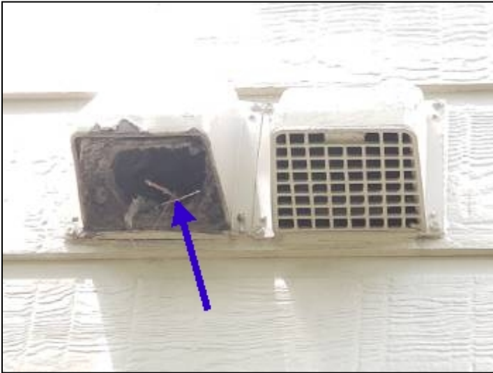
Indications are that there is a bird nest in one of the vents.
