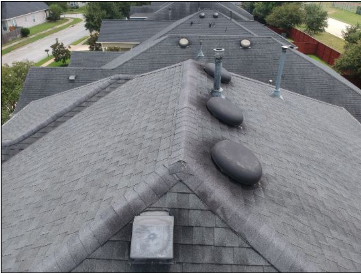
Overview of roof
