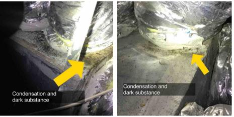
• The return filters located in the attic are dirty, the A/C system/coils need to be evaluated further and cleaned by a qualified HVAC contractor to check for possible damage/rust issues, units need to be cleaned and filters need to be replaced and ducts should be evaluated for cleaning also.
