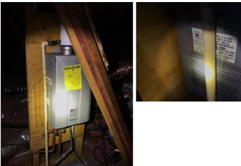
TPR - Not Tested: The temperature and pressure relief (TPR) valves are not tested/operated due to the potential for leakage
