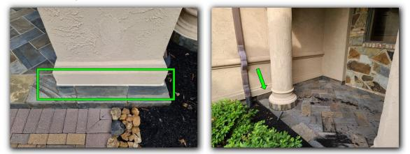
Sealant was present at the visible kickout / diverter flashings. The sealant should be maintained.
