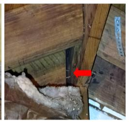
• There is no support beneath ridge board joint. Recommend further evaluation and repair as needed by a qualified roofing contractor to prevent possible sagging of ridge.
