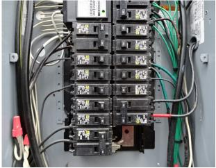
• The 50 amp circuit breaker labeled "A/C" is oversized for the equipment installed. Max breaker size should be 40 amp per the manufacturer. Repair by a qualified electrical contractor.
