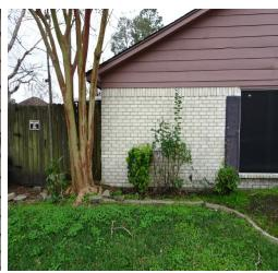
Soil is of reverse grade on multiple sides of the house (low spots, negative slope, etc), creating vulnerability to the accumulation of standing water at the foundation wall, a condition known to be a factor in foundation failure. Re-grading is required for a more positive drainage. Samples below.
