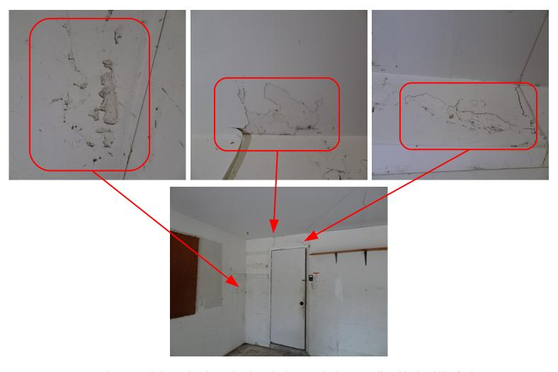
• Water damage and elevated moisture levels on both master bathroom walls. This should be further evaluated and properly repaired by qualified contractor(s).
