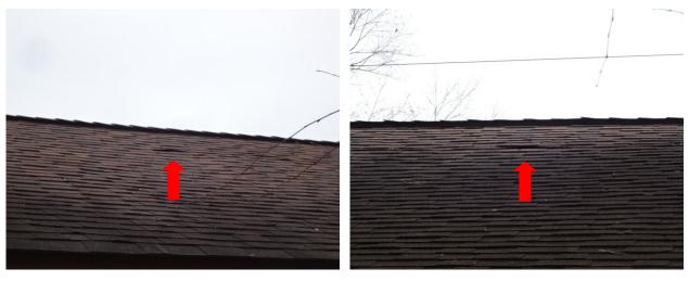
• Sags/depressions on multiple sides of the roof. This may be associated with structural movement. Recommend further evaluation and proper repair as needed by qualified contractor(s).
