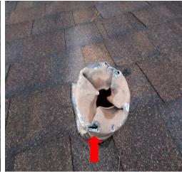
• Improperly installed chimney flashing. Repair by a qualified roofing contractor to prevent premature deterioration and possible water intrusion.
