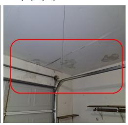
• Repaired water stains at in multiple areas. Elevated moisture levels were not detected at the time of inspection (Moisture Meter: Flir MR: 60) Investigate root cause and confirm that all affected areas such as but not limited to: sheetrock, insulation, joists, etc, have been properly repaired/treated by a qualified contractor. Note: If not properly repaired and or treated, it can lead to microbial growth.
