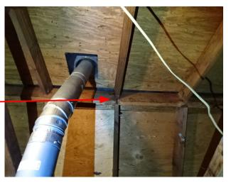
• Observed absence of "H" clips between sheathing **Note:** H-clips increase panel stiffness by allowing distribution of weight between adjacent panels.
