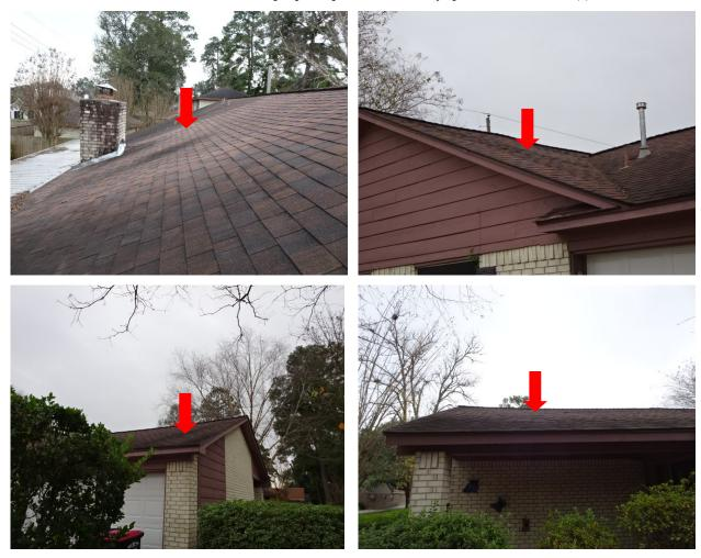
• Damaged lead pipe boots on multiple plumbing vents. In need of repair by a qualified roofing contractor to prevent possible water intrusion and damage to property.
