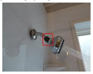
• Water/foreign substance and oxidation on the hallway bathroom shower plumbing visible in through the attic access. Recommend further evaluation and repair as needed by a qualified plumbing contractor.
