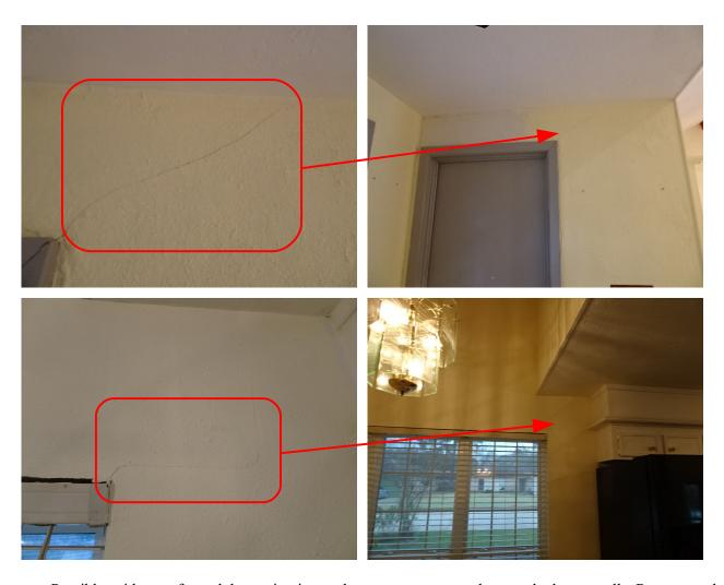
• Possible evidence of wood destroying insect damage on garage and master bedroom walls. Recommend further evaluation and treatment as needed by a qualified pest control contractor.
