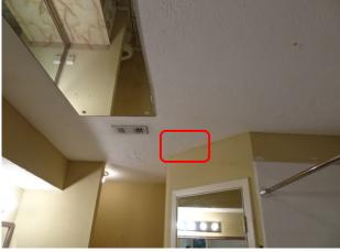
• Evidence of microbial growth on the hallway bathroom ceiling. This may be caused by improper ventilation of the bathroom. Further investigate root cause and properly repair and/or treat as needed by a qualified contractor(s).
