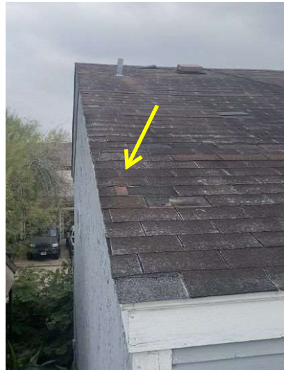
Missing shingles
