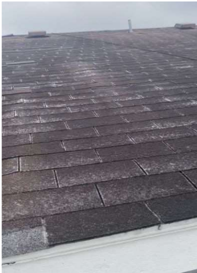
Older roof - less grains left of shingles
