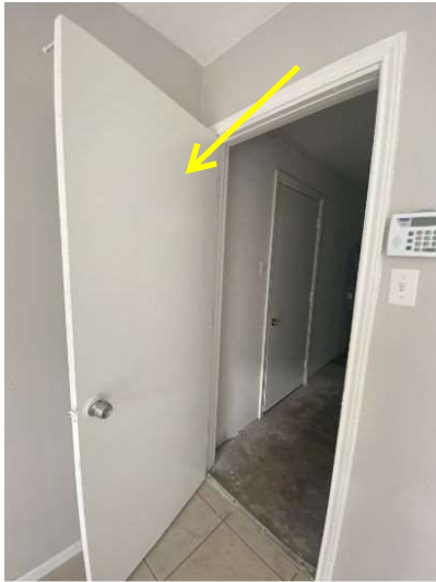
No solid/ fire resistant door installed at garage to house entrance
