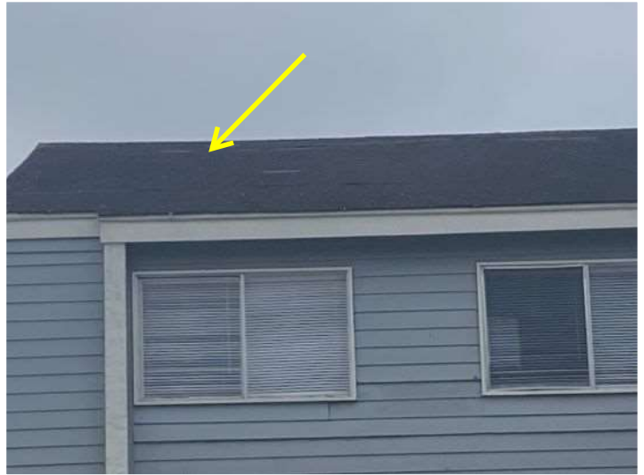
Missing shingles
