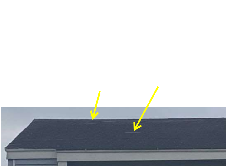
Missing shingles
