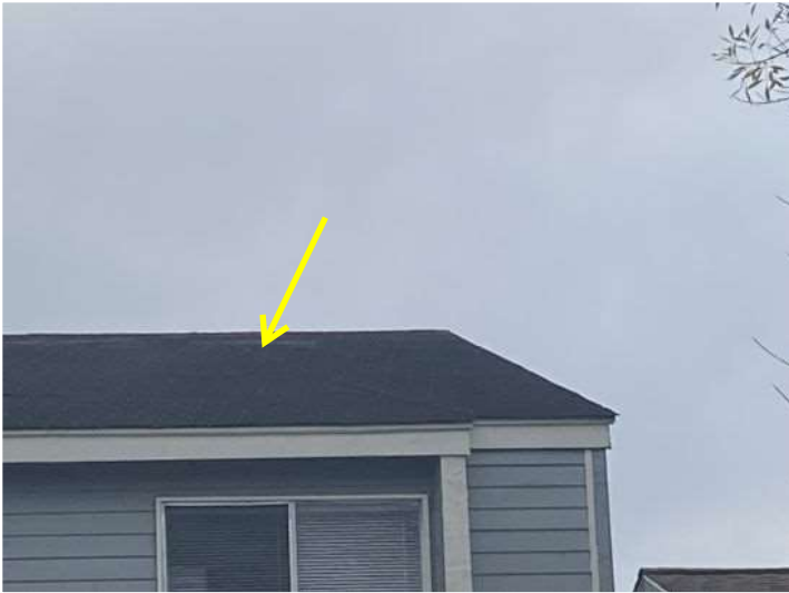
Missing shingles
