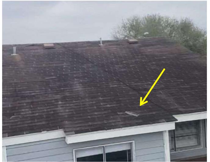
Missing shingles
