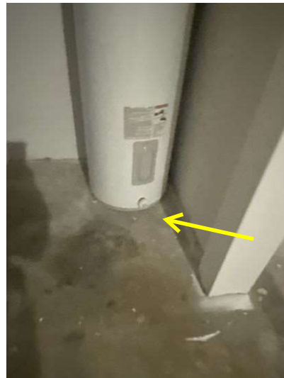
Water heater should be placed 18 inch above ground when installed in garage
