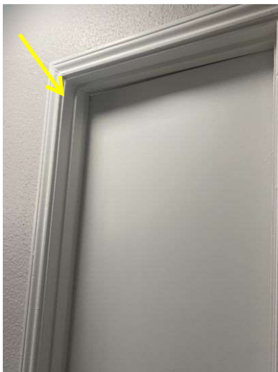
Door jamb in frame -bedroom upper level , 2nd bedroom
