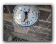
Static water pressure is required to be between 40 and 80 psi. Pressure below this range may result in fixtures an/or appliances that do not function properly. Higher pressure may reduce the life of installed plumbing, fixtures and appliances.
