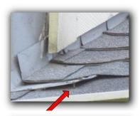
5. Observed various nails backing out of roofing material. Recommend replacing with new nails and properly sealing the area.
