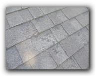
7. The entire roof system shows some signs of aging. However, the roof was performing as intended at the time of the inspection.
