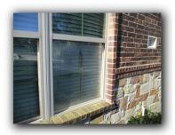
34. Observed what appears to be the hermitic seal for various windows may be starting to fail. Although the seal could be still intact, there is no way of determining when or if it will completely fail. Recommend having a qualified window company examine and repair all issues.
