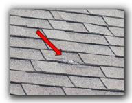
8. Broken or damaged shingles were noted on roof area.
