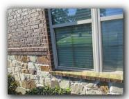
33. Window screens were noted that are either missing or torn. Screens are mentioned in this part of the report as they are a specific item in the T.R.E.C. guidelines. Screens that are torn enough to allow insect infestation should be repaired. All windows and sliding glass doors that have channels for screens should have them installed.
