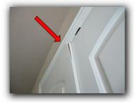
27. Observed damaged door, not closing. Recommend replacing or repairing door.
