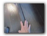
36. Observed areas of flooring material on the stairway that appear to be a trip hazard.
