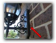
43. Recommend caulking and sealing exterior light fixtures. This will help prevent possible insect infestation and moisture penetration to the structure.
