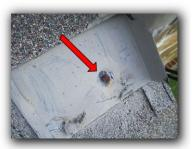
9. Exposed nail heads at either the vent & roof flashing or at the composition shingles can allow water to penetrate past the roof covering given enough time. As the exposed portion of the nail rusts, more space will become available between the nail and the roofing material for water to penetrate. This condition can usually be remedied by sealing or caulking affected areas.
