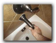
54. Shower hardware in loose in various locations. Recommended having it tightened up to prevent water penetration into the structure.
