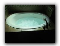
63. Hydro-therapy tub does not have a readily accessible inspection port. The pump equipment should be checked on a regular basis for leaks. The absence of an inspection port reduces the ability of an inspector to adequately determine the condition of the equipment.
