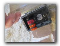
41. Observed an absence of GFCI (ground fault circuit interrupter) protection in required locations.
