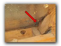
14. Observed some wood rot in various location in the attic. any wood rot and or decayed wood should be replaced or repaired. By replacing or repairing you prevent wood destroying insects from invading the wood and causing further damage.
