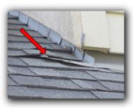
12. Roof flashing is loose or damaged in various areas. This condition is considered to be a conducive condition for water penetration and can be uplifted in high winds. Sealing and securing the flashing is recommended.
