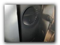
38. The flue has creosote and/or soot build up. Recommend having a chimney sweep check and clean the system before using.
