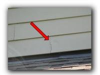
16. Observed some damaged siding or trim. Recommend replacing all damaged areas to help prevent possible water or insect penetration to the structure.
