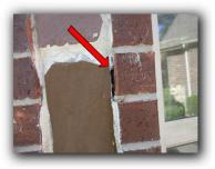
17. Observed areas of mortar shrinkage. This is common on stone or brick veneer homes. As the mortar dries, it will begin to pull away from the material. Recommend pointing up these areas with mortar or sealing with a proper exterior sealant.
