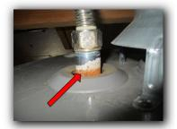
62. Observed corrosion/rust at water heater plumbing connections. Repair/replace plumbing connections as needed
