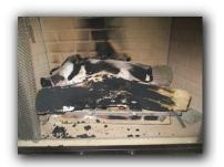
37. Observed buildup of soot on ceramic logs in fireplace. This could be the result of improper combustion, or the logs may not be in the proper position. Consult fireplace specialist.
