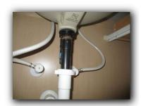
57. Observed leaking drain under master bathroom sink. These leaks can promote water penetration to the structure. Concealed damage is a possibility. Recommend having a licensed plumber repair the issue.
