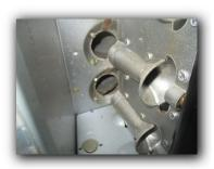
49. Burners rusty and dirty; recommend service by heating company to check for proper operation.
