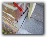
11. Roof penetration(s) not properly flashed/sealed. Recommend repair by a licensed roofer.
