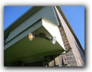
44. Some lights did not function when tested. Light bulbs should be replaced and fixture operation verified to ensure an underlying electrical problem does not exist.
