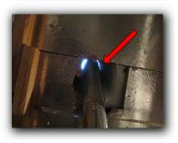
10. Missing sealant on rain skirts on metal fireplace or furnace flues. Recommend sealing skirts to help prevent against water penetration.
