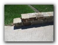
39. Observed damaged and loose deco-stones at entry to driveway. Recommend repair by a qualified contractor.
