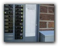
40. The circuit breakers are not identified and labeled. Proper labeling of circuit breakers can be crucial during an emergency situation.
