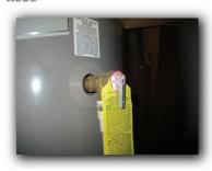
61. The temperature and pressure relief valve did not function when tested.
