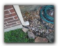
3. Missing splash plate for the guttering system in various location.
