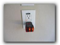
42. GFCI (ground fault circuit interrupter) not tripping when tested with external device in garage
