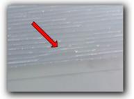
6. Observed areas of raised or lifted shingles. Recommend having these areas properly nailed down and sealed to prevent damage in high winds.
