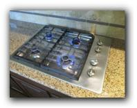
67. Igniter not functioning for burners, indicators are worn away.
