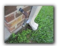
65. Gas outlets are not connected to an appliance. These should be capped gas tight.
