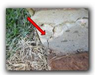
2. Corner cracks were noted on foundation. It has been noted that cracks in the outside corners of the perimeter beams are caused in many cases by the shrinking of the concrete in the perimeter beam as it dries and the rigidity of the brick and mortar against this drying process. It is normally not an indication of foundation failure or the need for foundation repair.
