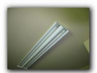
47. Observed various globes/covers missing from light fixtures. This is a recognized safety hazard.
