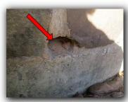
19. Weep holes are to large. Weep holes should be no more than 5/8" holes, current size may let in pests.
