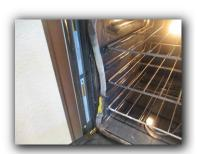
68. Gasket is damaged on oven door, door does not appear to seal properly.
