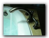
55. Master tub fixture does not spray properly. Recommend cleaning or replacing screen.
