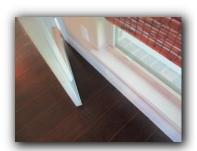
26. Door stops are missing,damaged or need repositioning in various locations. The installation on of door stops on all interior and exterior doors to help avoid damage to walls and door hardware is highly recommended.
