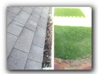
4. Gutters have leaves, limbs and other debris located in them. Periodic cleaning of the guttering system is recommended. I=Inspected NI=Not Inspected
