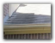
13. Observed extensive deflection in roofing materials. Roof should be further evaluated and repaired by a licensed roofer.
