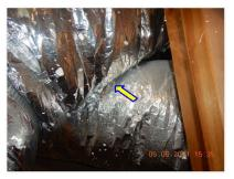
☑ Separate ductwork where touching at attic to prevent thermal bridging. Thermal bridging causes condensation to form between the duct lines and can drip into the attic. LEAKS and AIR FLOW: **NI=Not Inspected**
