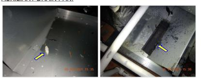
☑ Insulation/debris observed at the A/C auxiliary condensate drain pan.
