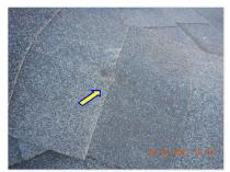
☑ Excessive aggregate loss observed at ridge cap shingles. FLASHINGS:
