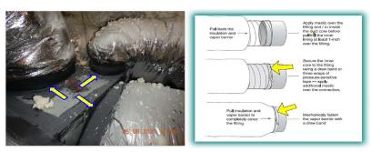
☑ Mastic has been applied to the outside of the ductwork. Normally, the inner ductwork liner should be sandwiched between two layers of mastic.
