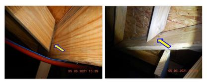
☑ Rafters cuts not flush at the ridge, hip and or valley boards in the attic. *Attic Moisture Deficiencies:*
