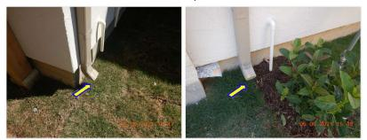
☑ Splash blocks should be placed in areas where water can accumulate near the foundation edge. The discharging of the rainwater from the gutters needs to be directed away from the foundation edge.
