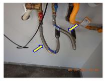
☑ Hot and cold water lines should be insulated within 5' of the unit.
