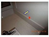
$\square$  Caulk missing or deteriorated around the sink counter area at the following locations: Master bathroom.
