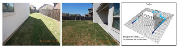
The drainage and grading around this home is inadequate. In order for the drainage to be effective, the landscaping must be configured so that the yard is sloped away from the foundation by at least 6 inches in the first 10 feet and/or adding additional gutters/downspouts to the house is another option to improve drainage and/or in- ground drains should be designed and added to divert rainwater and runoff away from the house as appropriate and/or drainage swale should be improved/installed.
