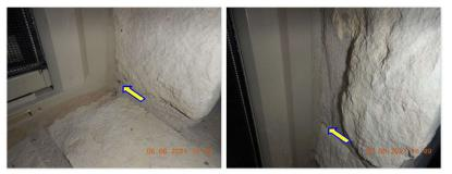
☑ Caulking around exterior windows deteriorating.
