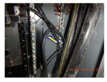
☑ The black insulated conductor used for grounding and or bonding should be marked green. *Service-Entrance Equipment Grounding and Bonding:*
