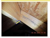
☑ Rafters were secured to the ridge board with 0 nails on one side, versus the appropriate number on one side, the appropriate number on the other.
