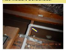
$\square$  Insulation is missing on the condensate drain line and/or water lines in the attic. The water and drain lines should be completely insulated in the attic.
