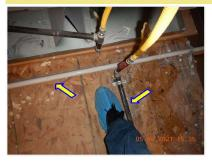
$\boxdot$  Gas pipes and/or wires and/or water lines are crossing directly over the top of the attic service walkway.
