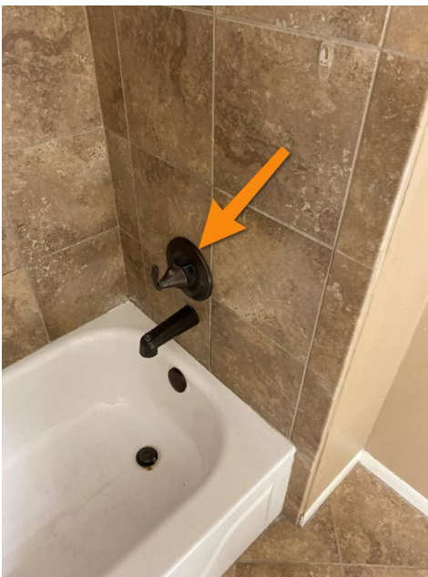
2nd Floor Bathroom
