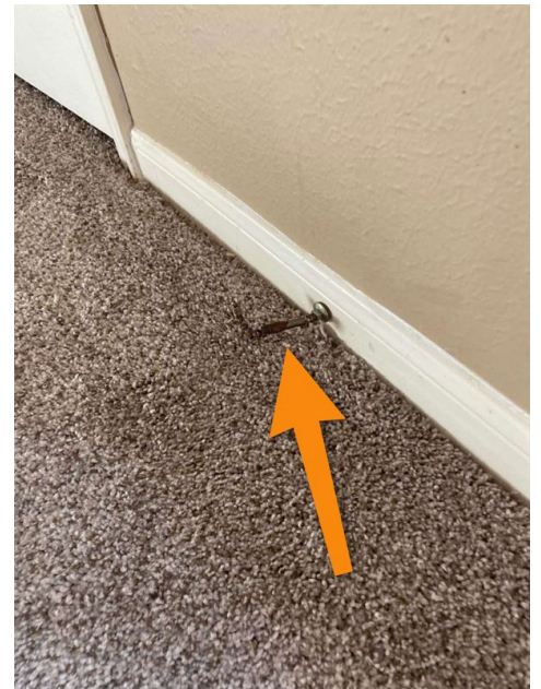
2nd Floor Hall
