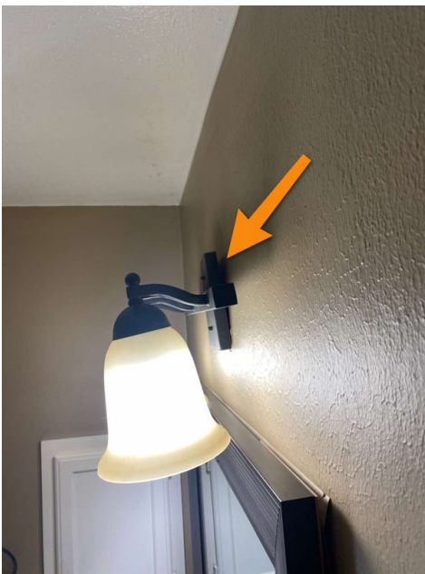
2nd Floor Bathroom
