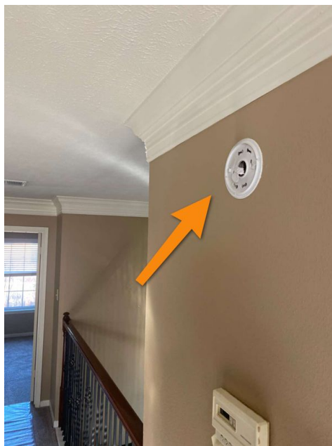
2nd Floor Hall
