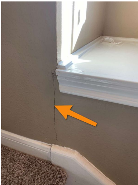
2nd Floor Hall
