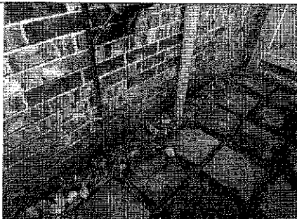
Ground Rod Not Visible
