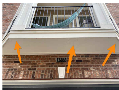
In front of garage.
