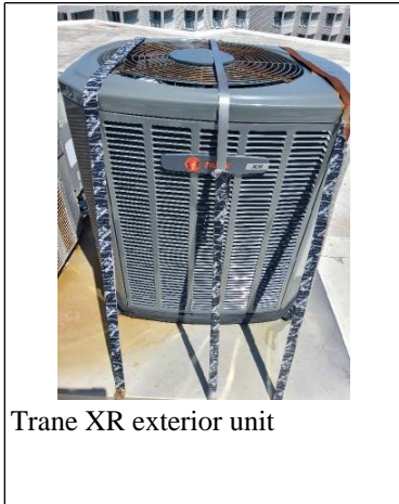
Trane exterior unit manufactured in 2019, rated at 2 tons, and uses the newer refrigerant R410A
