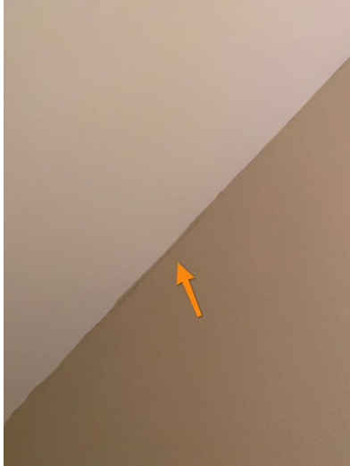
1st Floor Hall Bathroom
