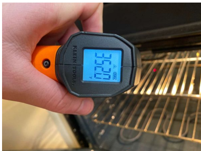
Photo(s) of 2nd oven: Kitchen
