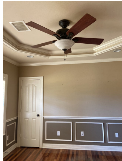
Ceiling fan in guest room not operating
