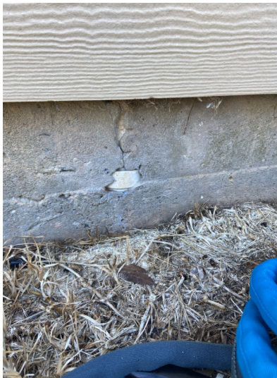
Pipes visible in foundation wall
