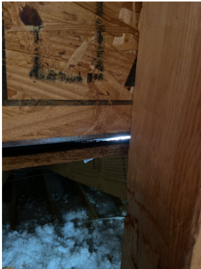
Light can be seen coming under roof flashing in attic. Should be sealed
