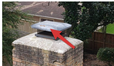
Rusted chimney cap
