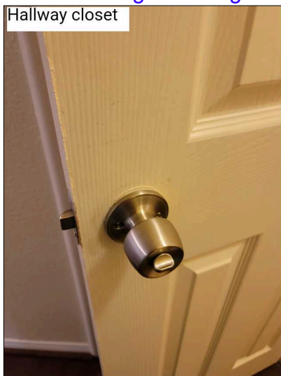
Several closet doors have privacy locks installed backwards. Possible entrapment hazard.
