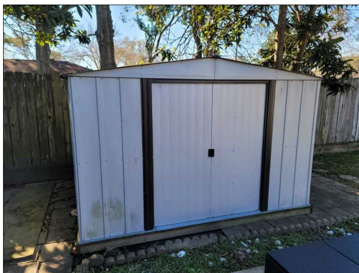
Outbuilding fully excluded from this inspection.
