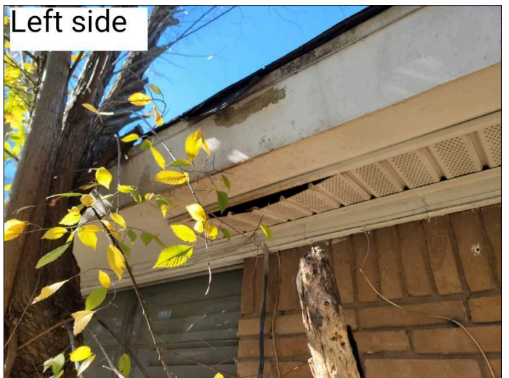
Open holes noted at edge of attic space. These could be a location for rodents to enter.
