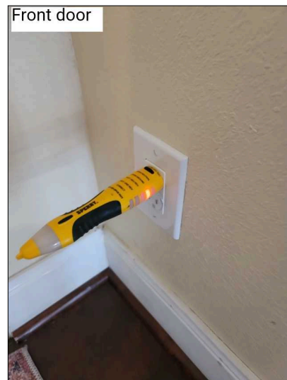
Numerous outlets tested as "Open Ground" These plugs should be evaluated and corrected / replaced.
