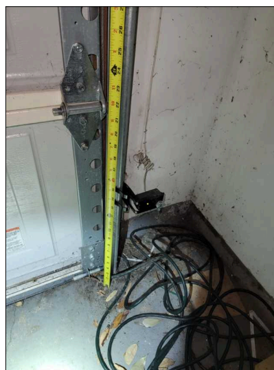
Opener sensing eyes higher than 6" above floor level.
