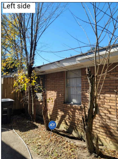
Trees in contact with house eaves. Suggest tree trimming to avoid damage.
