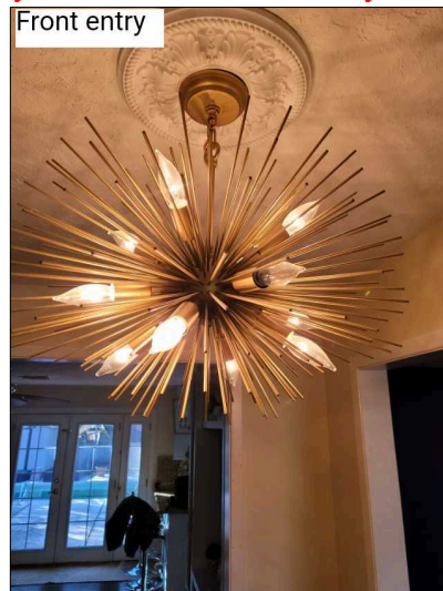
Fixture hangs too low, can hit a person walking in front door. Bulb out.
