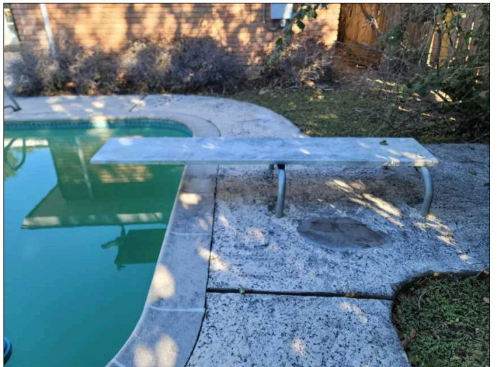
Diving board noted. Pool depth appears shallow for diving. Diving boards can increase the risk of injury or drowning if pool design is improper.
