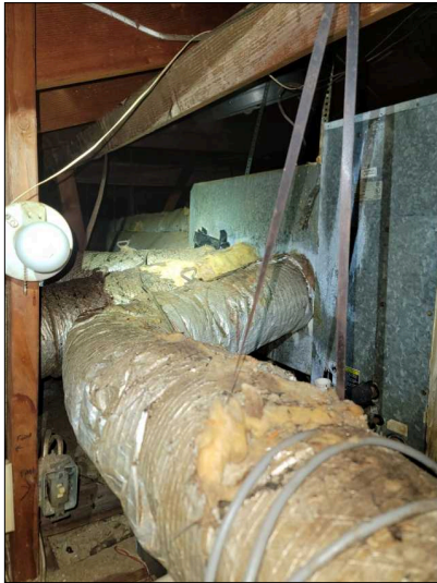
Rigid metal ducting present. This ducting is insulated with fiber blanket.
