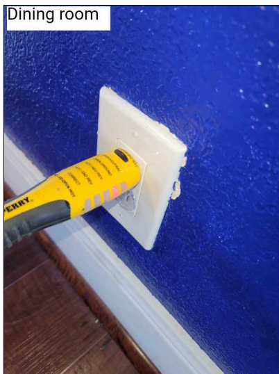
Numerous outlets tested as "Open Ground" These plugs should be evaluated and corrected / replaced.
