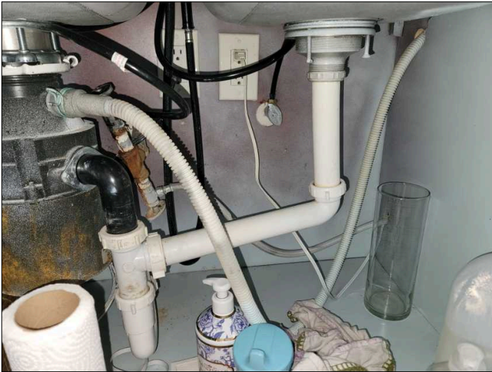
Drain line should create a trap by moving the flex drain line to the bottom of the counter top and securing.
