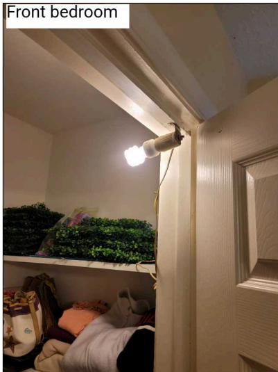
Open bulb light fixtures in closets are not allowed. Should be covered to reduce risk of fire.
