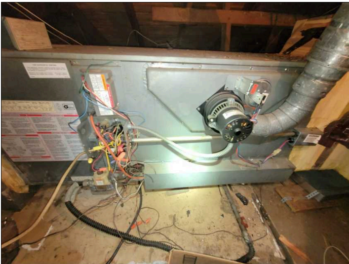
Access to equipment should have an open 30" x 30" landing to work, with 3/4" minimum decking.
