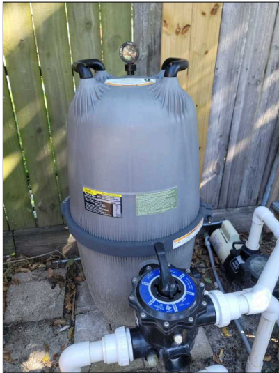
Diatomaceous earth (DE) pool filter. Follow MFR instructions when servicing. Use caution as DE can be harmful if inhaled or ingested.
