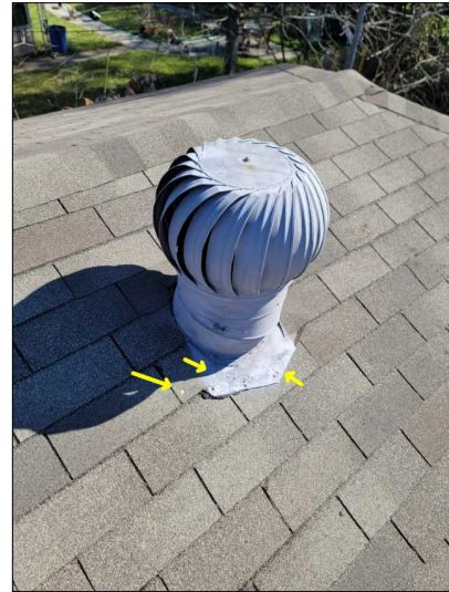
Exposed nails should be sealed over.
