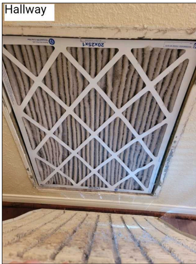
Change 1" filters every 30-60 days. Filter is dirty
