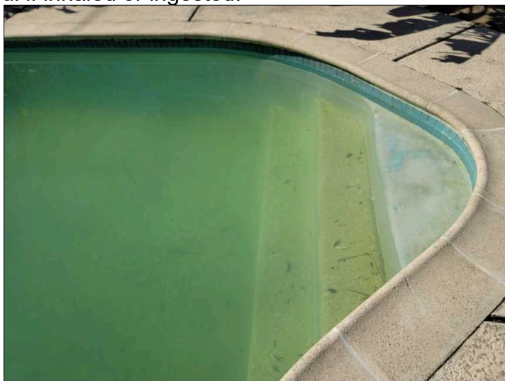
Pool water cloudy, dirty at time of inspection. Unable to determine condition of plaster, drains, jets, etc.
