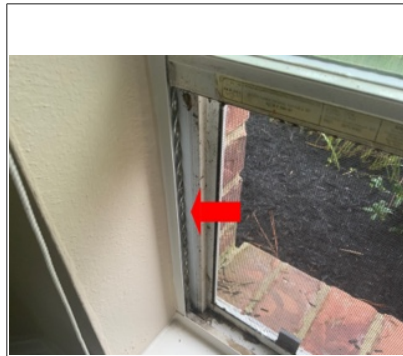
Sprung balance spring at dining area.
