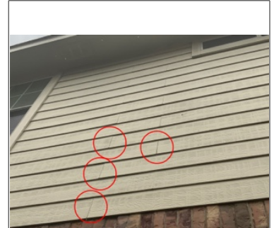
Siding seam separation at left of home.
