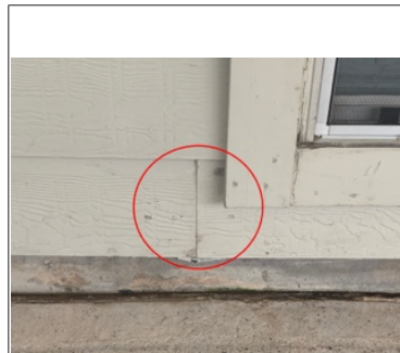
Trim board seal improvements needed at garage.
