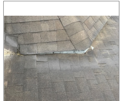
Seal all exposed nail heads.
