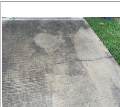
Driveway cracks.
