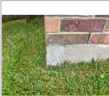
High soil blocking visual inspection of foundation at front of home.
