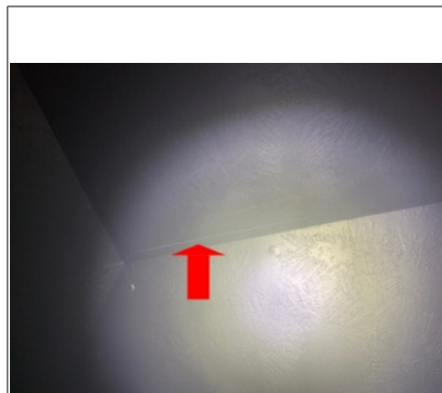
Seam failure at upstairs front left bedroom.
