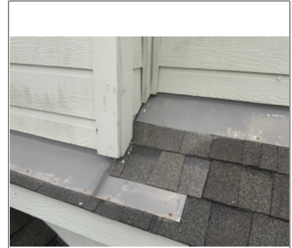
Seal all exposed nail heads.
