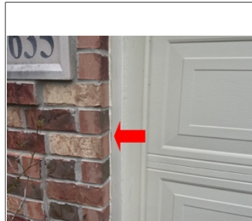
Minor settlement crack at entryway.
