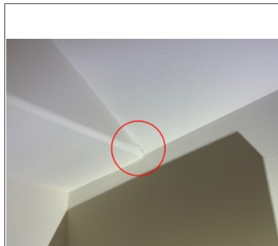
Seam failure at upstairs front left bedroom.
