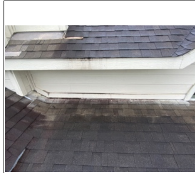
Flashing incorrectly installed.
