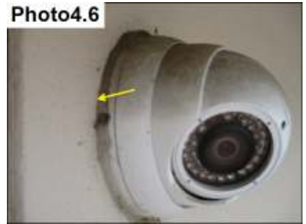
Penetration Sealants/ Seal
