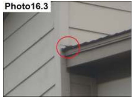
Roof Diverter Flashing Sealants/ Seal
