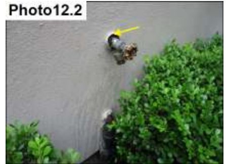
Penetration Sealants/ Seal
