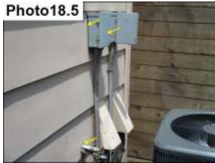
Penetration Sealants/ Seal
