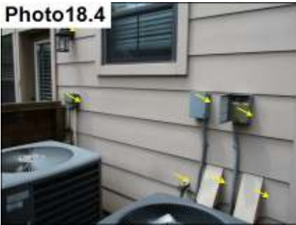
Penetration Sealants/ Seal
