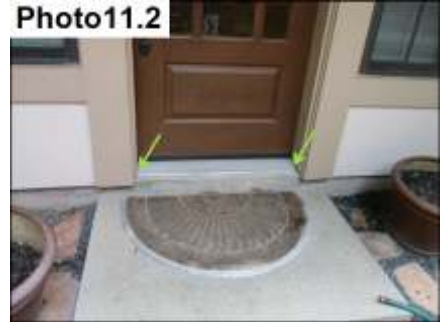
Door Trim and Miter Sealants/ Seal
