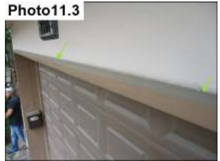
Door Trim and Miter Sealants/ Seal
