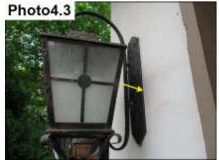
Penetration Sealants/ Seal
