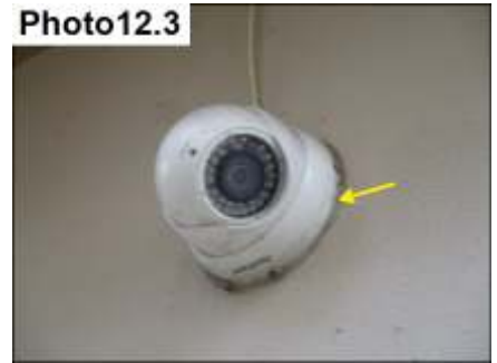
Penetration Sealants/ Seal
