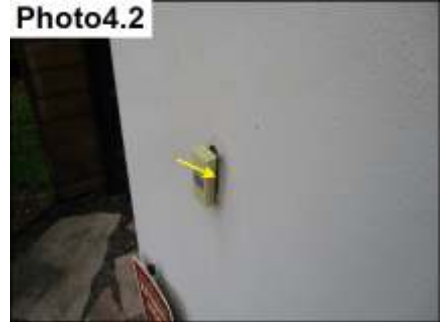
Penetration Sealants/ Seal
