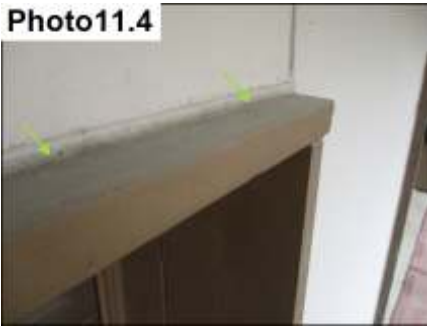
Door Trim and Miter Sealants/ Seal
