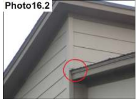
Roof Diverter Flashing Sealants/ Seal
