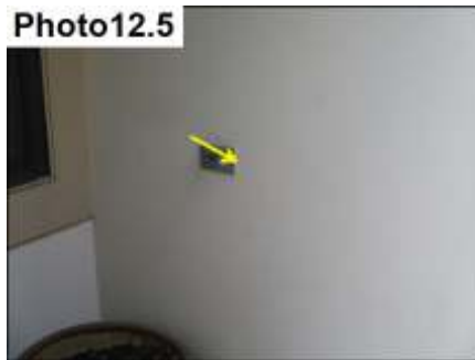
Penetration Sealants/ Seal
