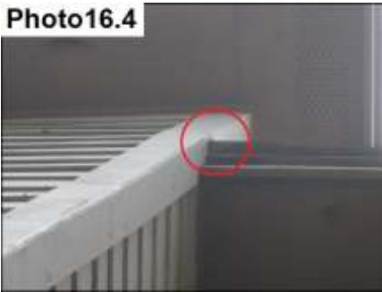
Roof Diverter Flashing Sealants/ Seal
