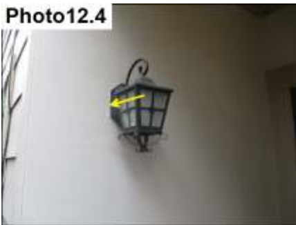
Penetration Sealants/ Seal
