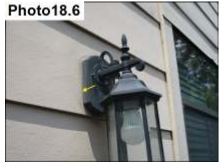
Penetration Sealants/ Seal
