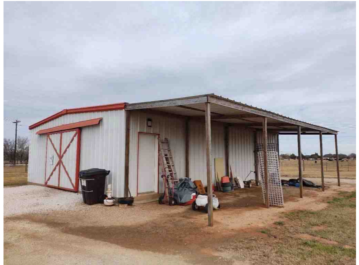
Metal Building Rear View
