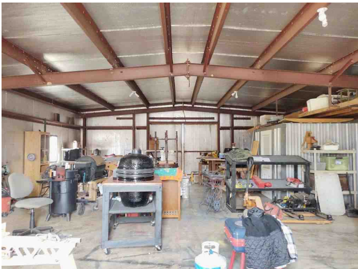
Metal Building Interior View
