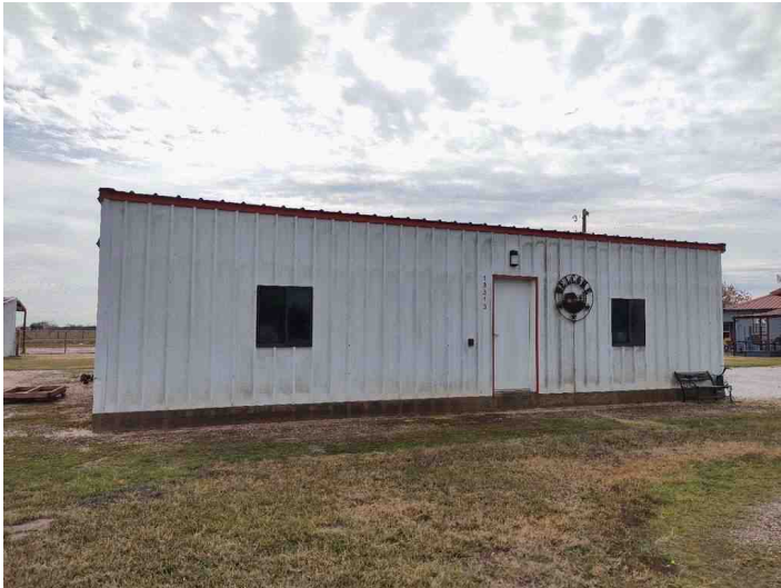
Metal Building Front View
