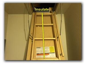
Did not observe a fire rating sticker on the attic access ladder in the garage. The sticker may have fallen off or has been removed. I could not verify that the wood for the attic access ladder has been fire treated as required by current standards.
