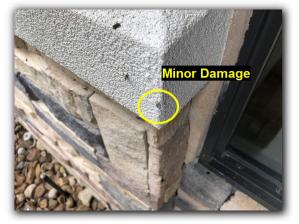
Recommend sealing/caulking around all holes, gaps, cracks and exterior siding penetrations to prevent water entry.
