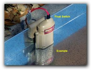
Recommend installing Safe-T-Switches on all condensate drain lines. This is not required, but highly recommended to help prevent flooding if the condensate drain line becomes clogged.
