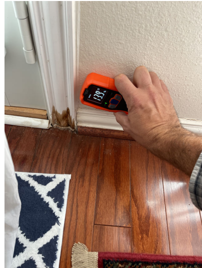
Moisture content acceptable at back door area
