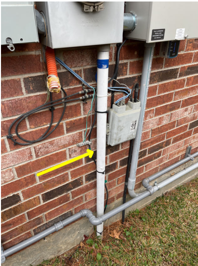
Support bracket needed
