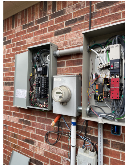
Overview of panels
