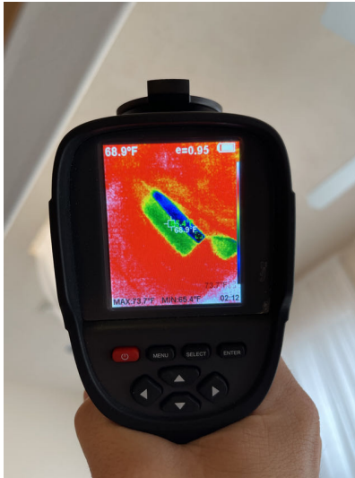
Thermal scan performed - no anomalies
