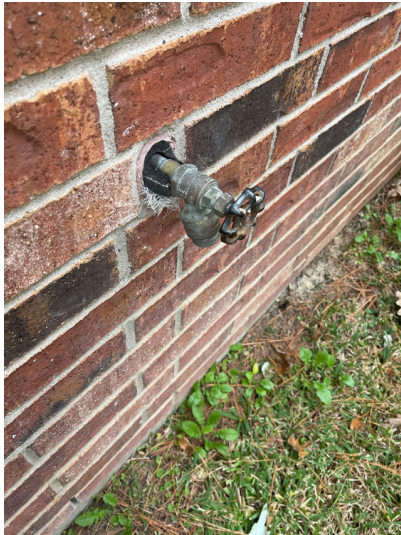
Insulation needed
