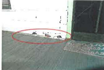
Several to the exterior siding tiles are cracked in spotted areas.
