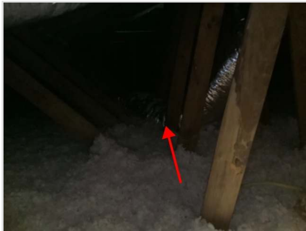
Inside attic space
