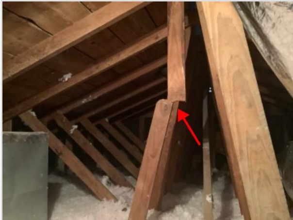
Inside attic space
