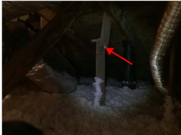
Inside attic space
