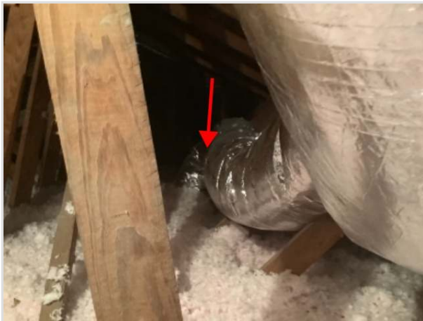
Inside attic space
