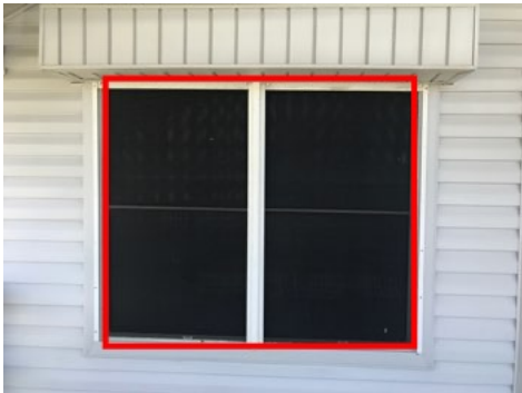
Around House: solar screens installed
