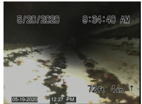
End of sewer scope at 72 ft
