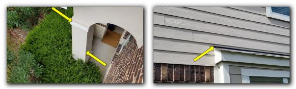
Install weep holes, required since 1992, at brick above lintels at maximum of 33" spacing above windows, entrance / exit jambs, garage overhead door jambs and elsewhere where lintels noted.
