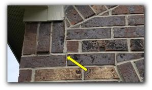
Area of deterioration/damage is noted at north and east sides of exterior siding and/or trim. All deteriorated/dmaged areas should be properly repaired and sealed, as needed, to prevent moisture penetration.
