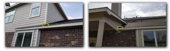
Numerous shingles, at lower south west side roof coverings, have lifting shingles and or lifting corners at shingles. All roof shingles that are lifting or have lifting corners need to be properly re-secured to lie flat, or need to be replaced and rechecked by manufacturer's representative, roofing contractor, or inspector for integrity and warranty.
