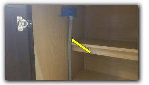
Properly secure flexible cable sheathing within 12" of J-box in kitchen island cabinet.
