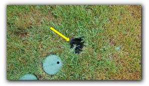
Sprinkler head noted at station 6 is noted as not working and is in need of repair/replacement.
